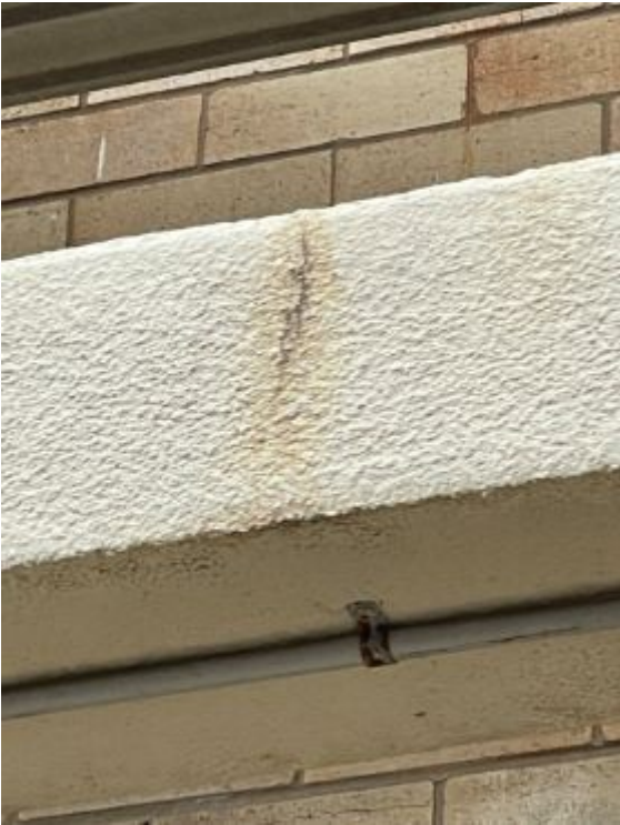
011 Existing Building Photos - Dated 26/09/2021
