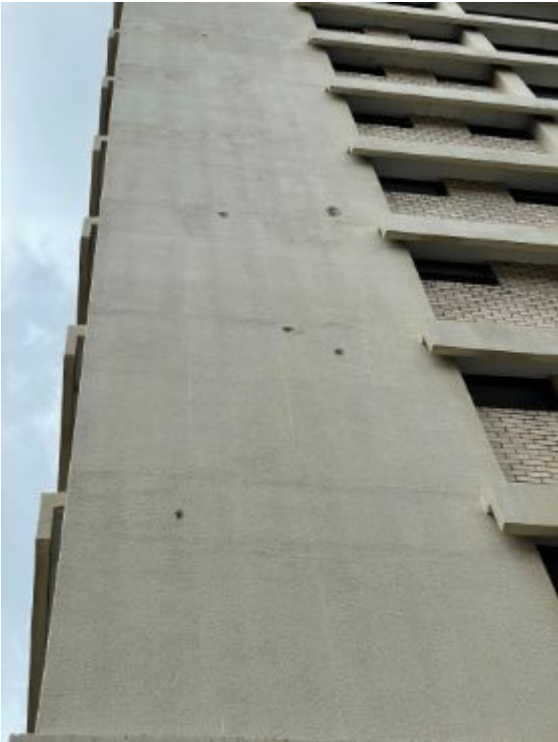
012 Existing Building Photos - Dated 26/09/2021
