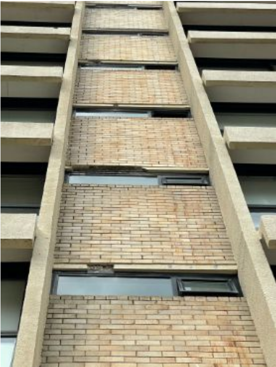
010 Existing Building Photos - Dated 26/09/2021
