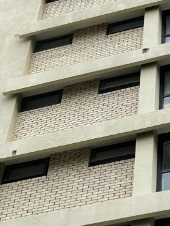
003 Existing Building Photos - Dated 26/09/2021
