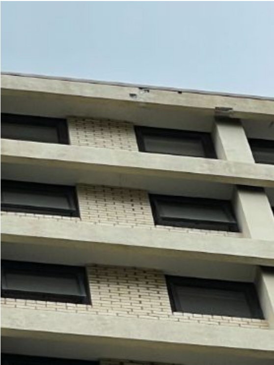
005 Existing Building Photos - Dated 26/09/2021
