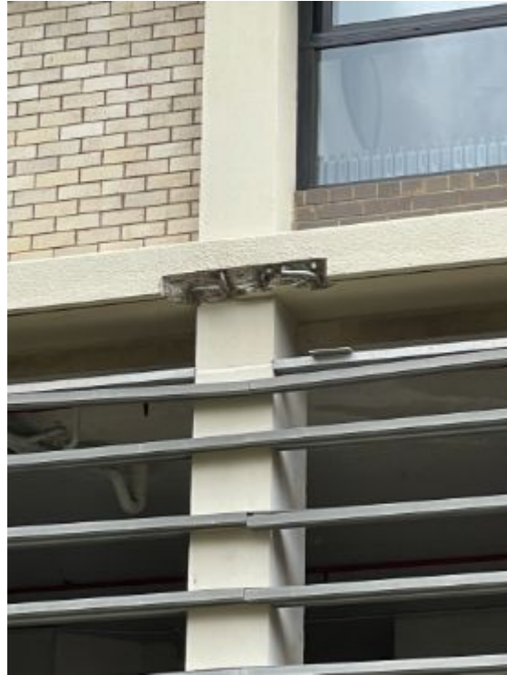
001 Existing Building Photos - Dated 26/09/2020
