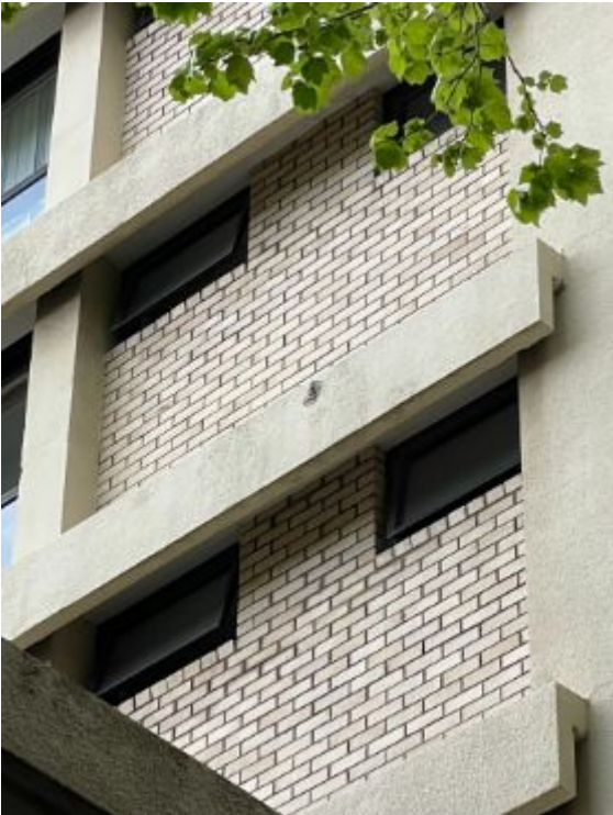
006 Existing Building Photos - Dated 26/09/2021
