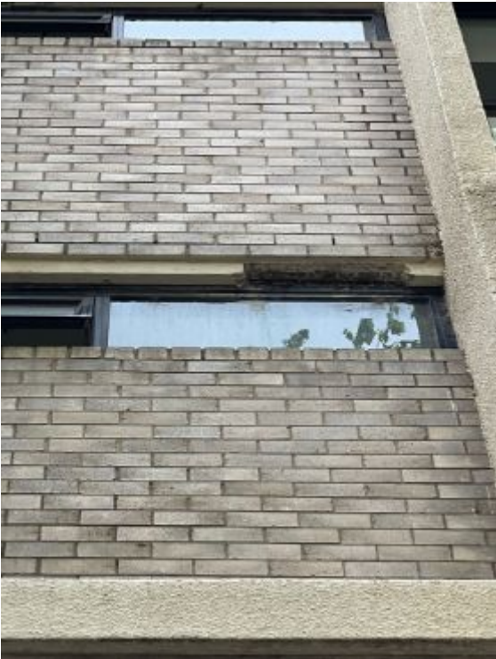
008 Existing Building Photos - Dated 26/09/2021
