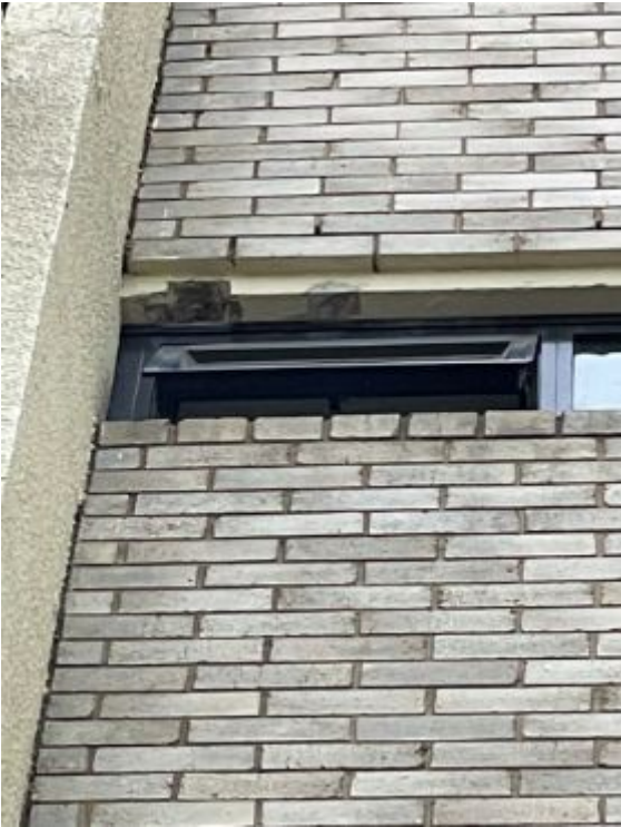
009 Existing Building Photos - Dated 26/09/2021
