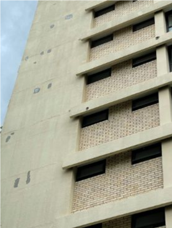
004 Existing Building Photos - Dated 26/09/2021
