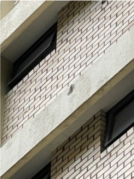
007 Existing Building Photos - Dated 26/09/2021
