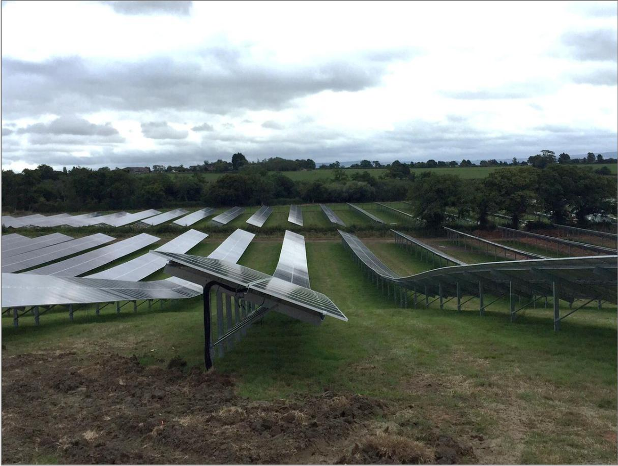
Figure 3-3: Fully assembled fixed array solar farm (image supplied by Infinergy UK)
