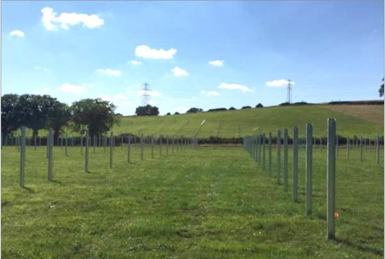
**Figure 3-1: Piles for the solar farm in place (image supplied by Infinergy UK)**
