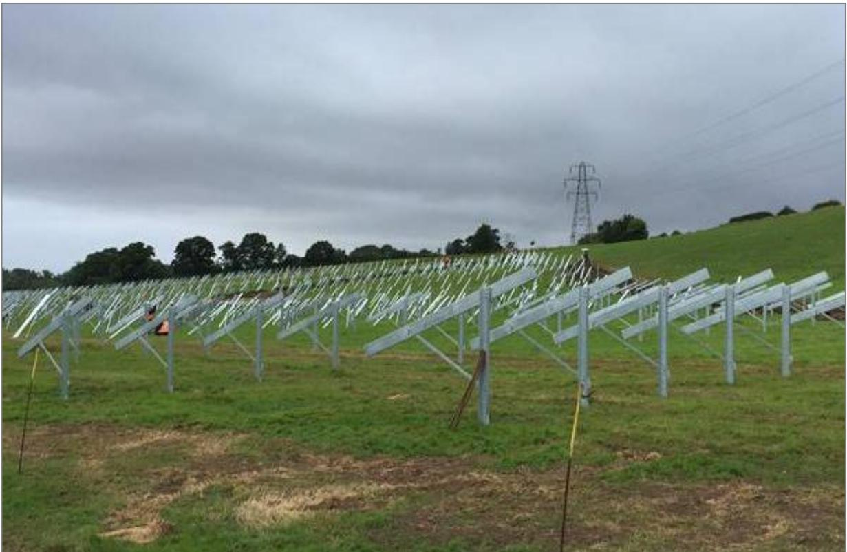
**Figure 3-2: Fixed array assembled before PV panels added (image supplied by Infinergy UK)**
