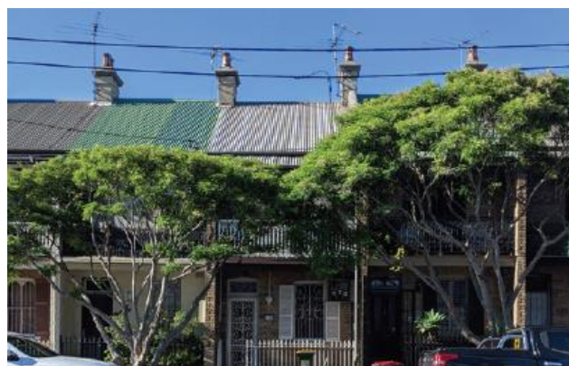
Picture 4 Existing residential properties to the south of Wellington Street
