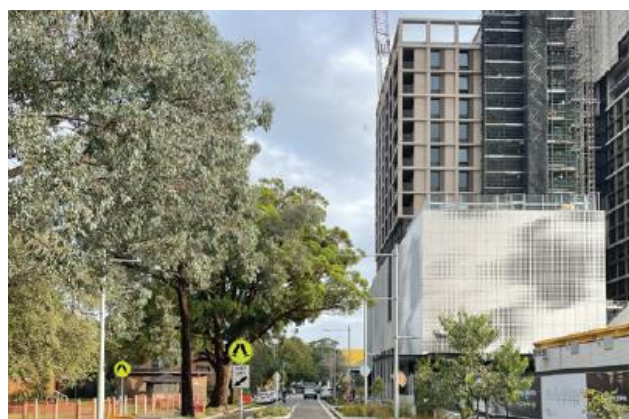
Picture 2 southern precinct (under construction)
