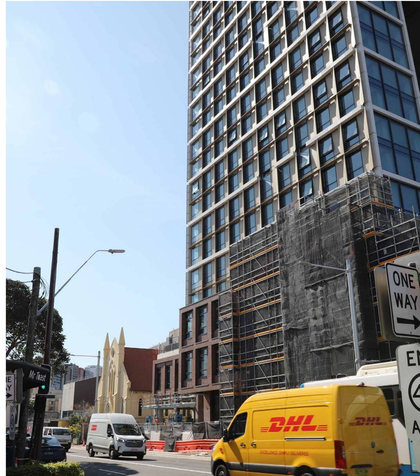
Photo 18. View north-west from the intersection of Buckland Street and Botany Road.
