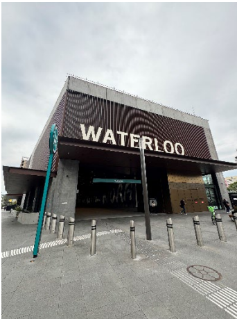
Picture 3 View of Waterloo Metro Station from Cope Street
