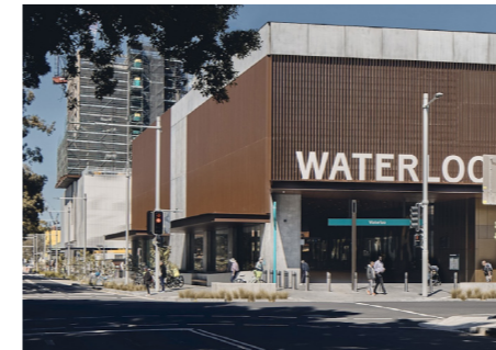
City of Sydney Light Poles
