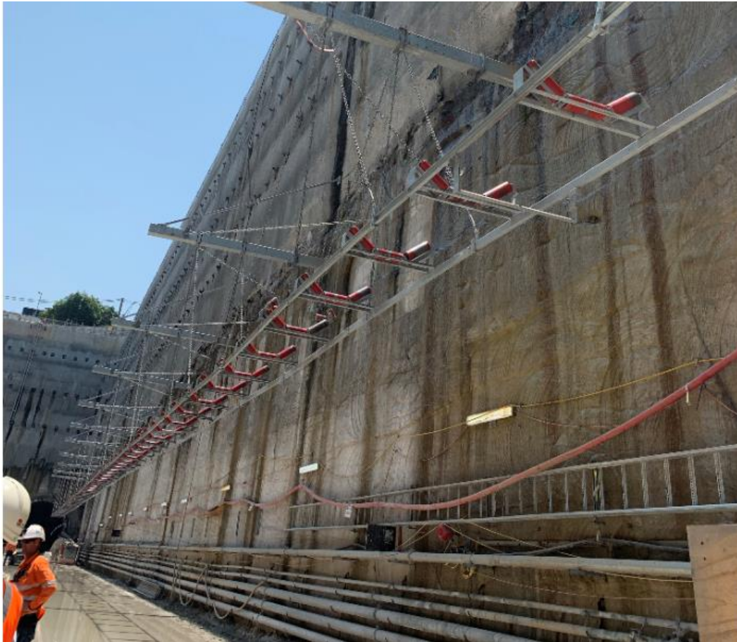
Figure 7.1 Exposed face of the excavation, depicting the Hawkesbury Sandstone formation
