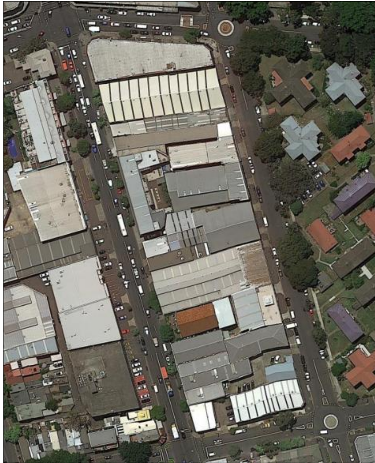
Figure 4.1 Aerial view of the site, pre-demolition of structures prior to the Sydney Metro and Waterloo Over Station developments, 2015 (Google Maps).
