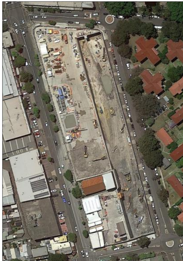
Figure 4.2 Aerial view of the site, post-excavation of the Waterloo Station Box, 2019 (Google Maps).
