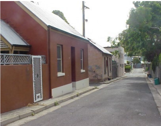
Figure 31 – View of Clarendon Street.
