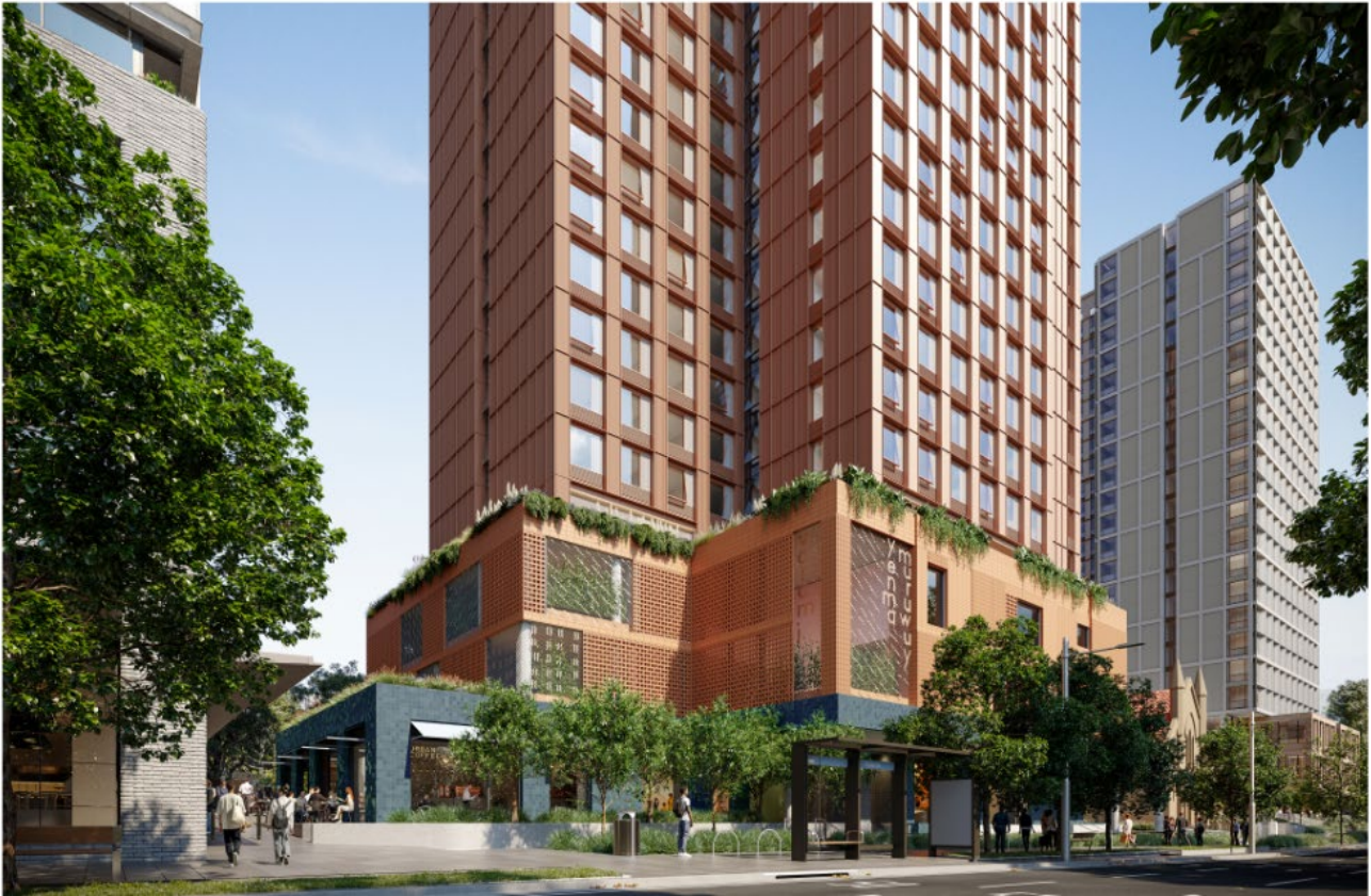
Figure 37 – Artist impression contained within the DA set showing the built form and the church (right).
