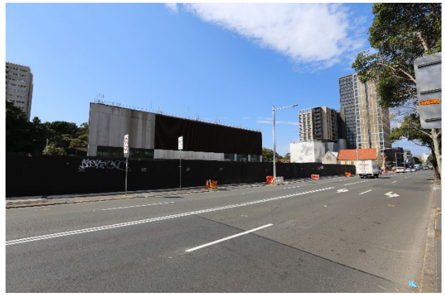
Figure 12 – East side of Botany Road, looking over the Waterloo Metro Quarter.
