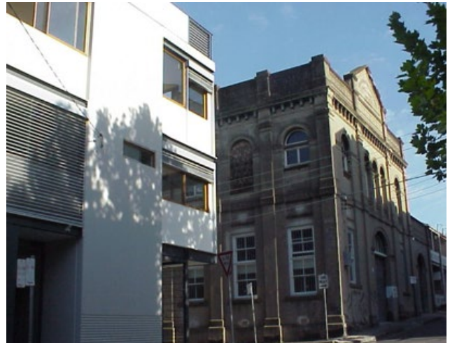
Figure 28 – View of Turner Street.
