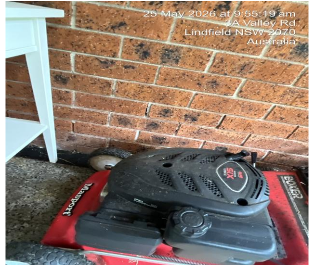
Photo 170 – Gaps observed to mortar
