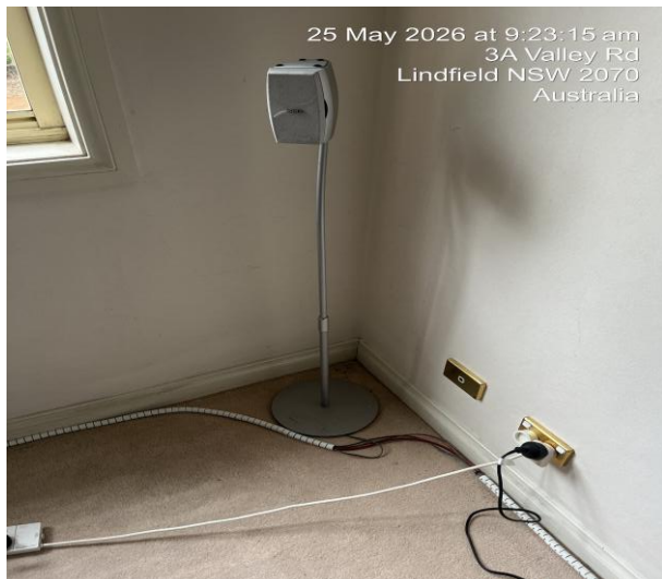
Photo 33 – Cracking observed to skirting
