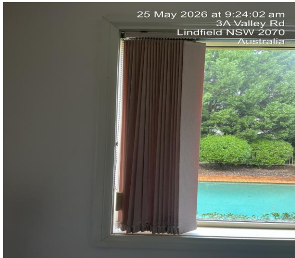
Photo 37 – Cracking observed to framing
