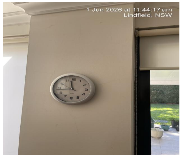
Photo 46 - Cracking observed to render
