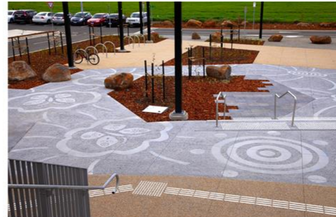
Ballarat Line Upgrade
