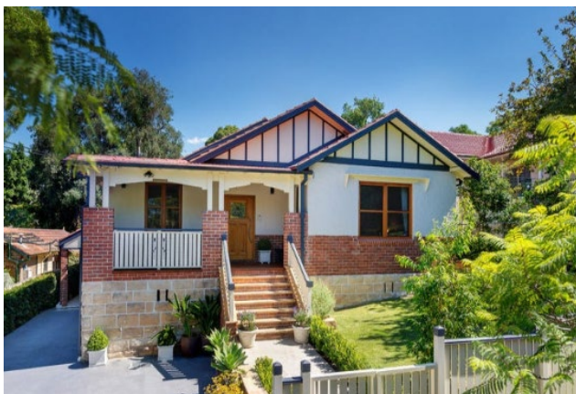
Figure 18: 52 Trafalgar Avenue, Lindfield to the west of the site (Realestate.com)
