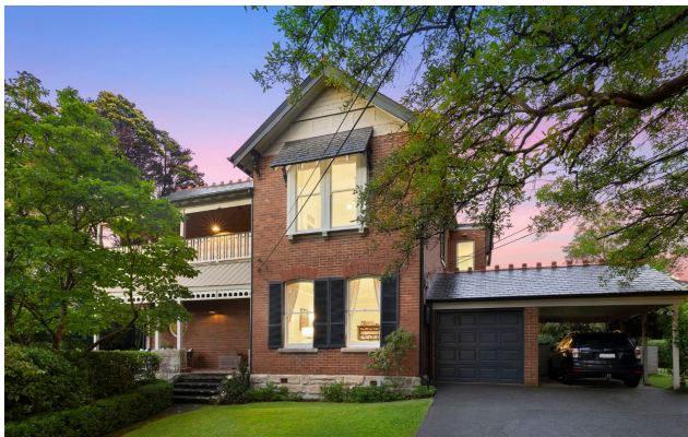
Figure 14: 1 Valley Road, Lindfield to the north, adjoining the site (Realestate.com)
