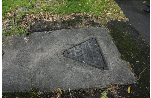
Figure 23 – Stormwater manhole locate on Woodside Avenue near No. 4.
