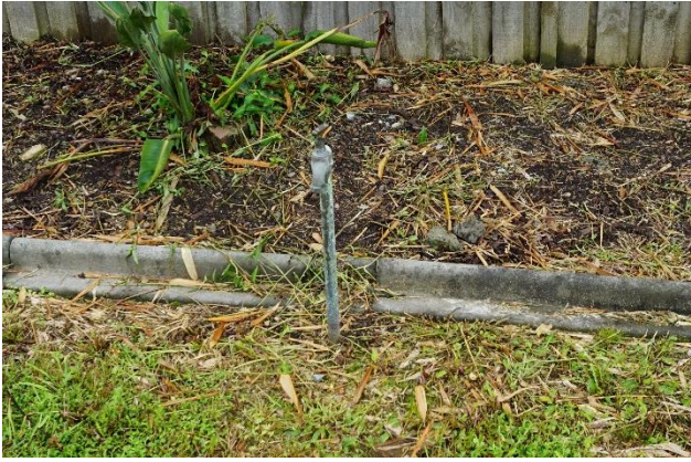
Figure 22 – Tap located in front yard at No. 4 Woodside Avenue.
