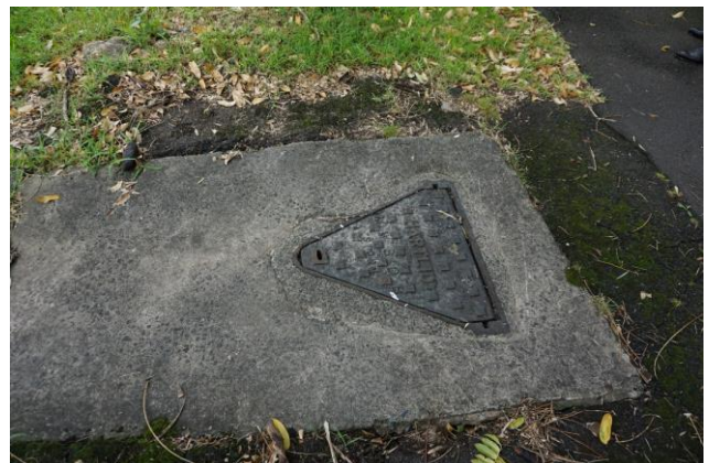
Figure 27 – Stormwater manhole located on Woodside Avenue near No. 4.
