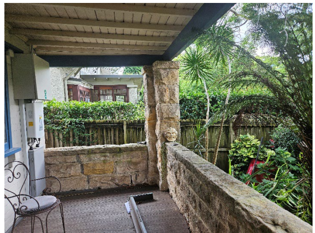
Figure 34 Front balcony – eastern view.
