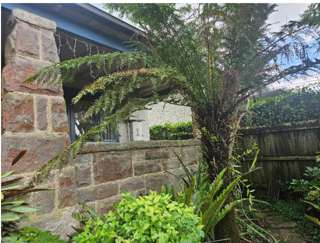
Figure 33 Eastern portion of front facade
