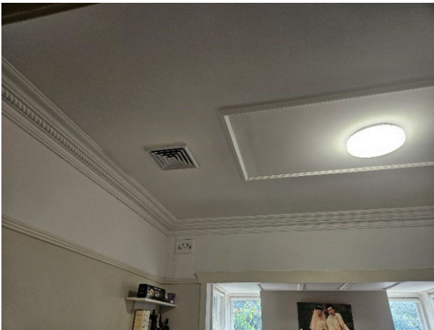
Figure 52 Ceiling detail with detailed cornice.
