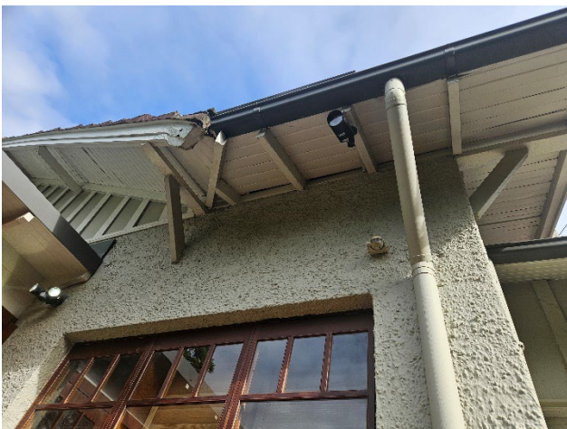
Figure 48 Extended eaves on roof gable.
