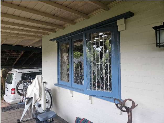
Figure 35 Western side of balcony with timber frame window.
