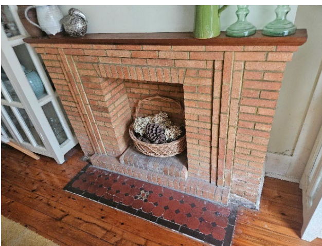
Figure 19 Brick fireplace original tiling to hearth.
