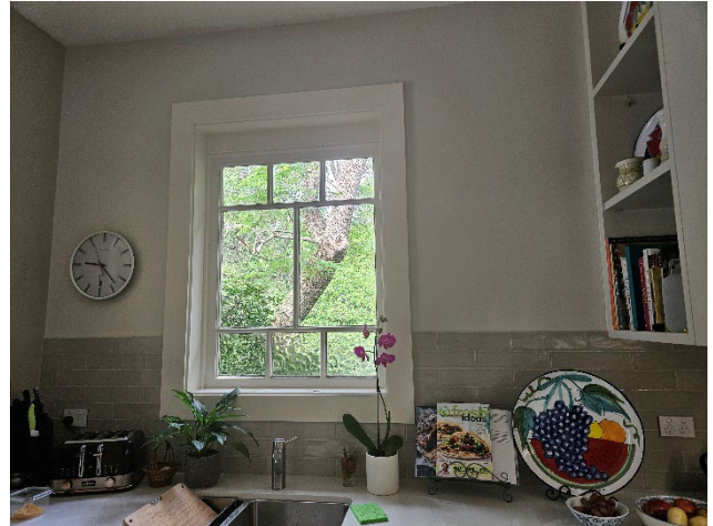
Figure 16 Interior view of original multipaned timber framed window located in kitchen area.
