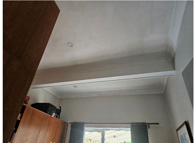
Figure 31 modified interiors with exposed ceiling beam.
