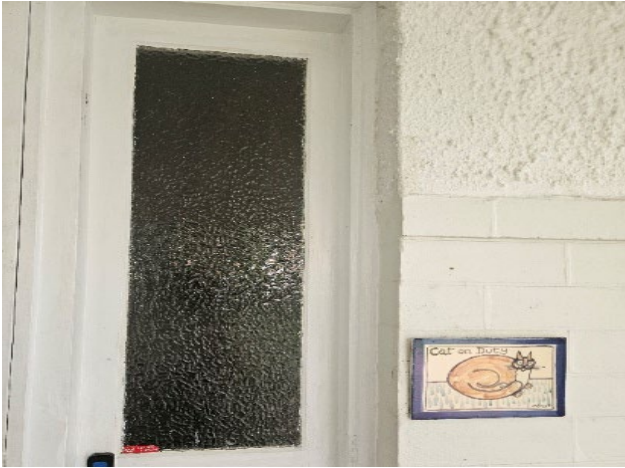
Figure 24 Single framed frosted window located to the front entrance.
