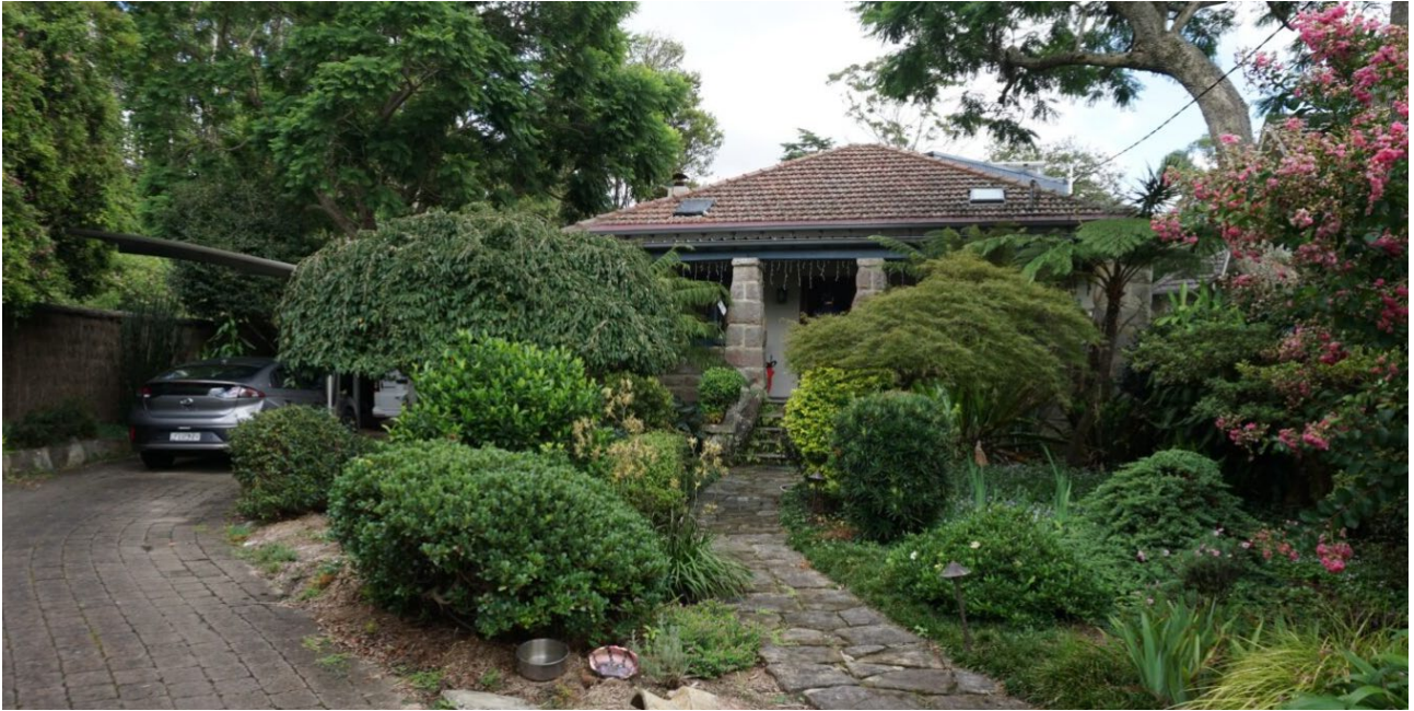
Figure 32 2 Woodside Avenue viewed from Woodside Avenue.
