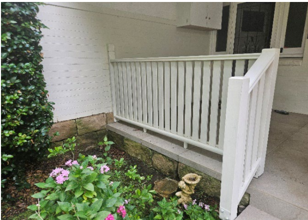
Figure 26 Balustrade located at front of the house.
