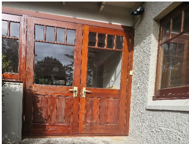
Figure 46 Front entrance – timber doors
