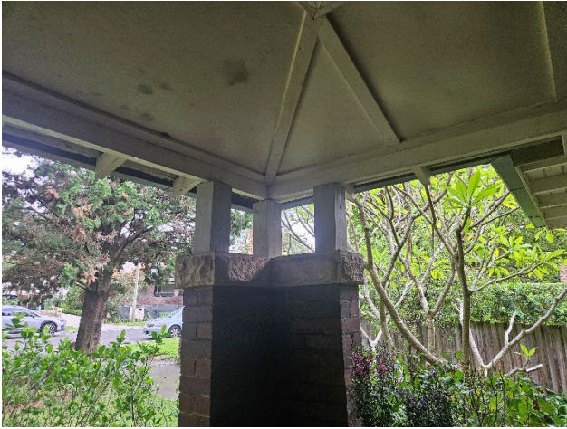
Figure 9 Front verandah roof timber detail.
