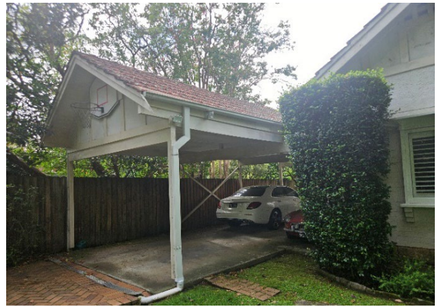
Figure 27 Extension carport adjacent to dwelling.
