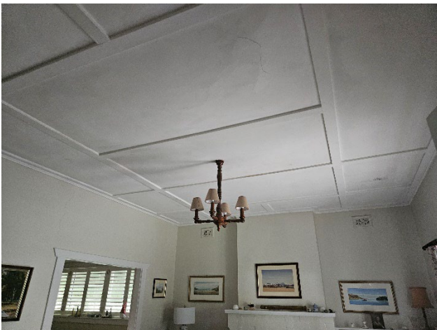
Figure 28 Modified interiors, original ceiling detail.
