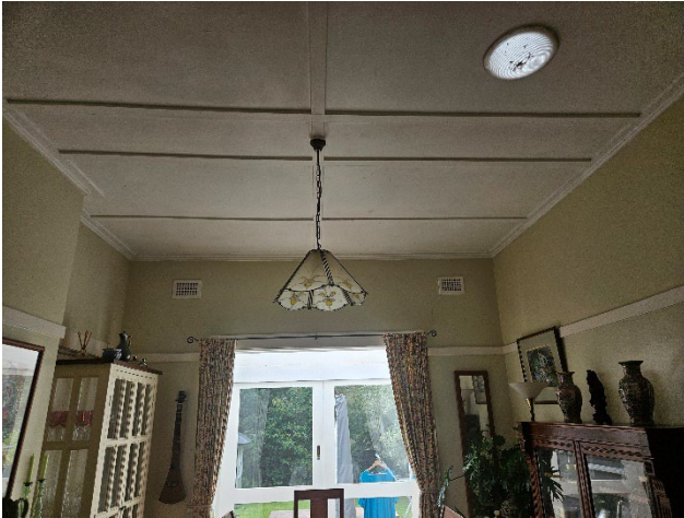
Figure 15 View of interior ceiling and picture rail on the wall.
