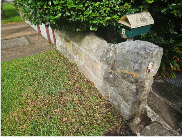
Figure 44 Sandstone fence on the southern boundary.
