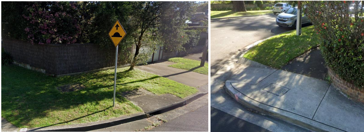
Figure 4. Existing manhole (left) and pit (right)
