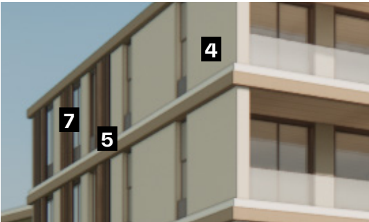
Texture rendered external walls in light sand colour.
