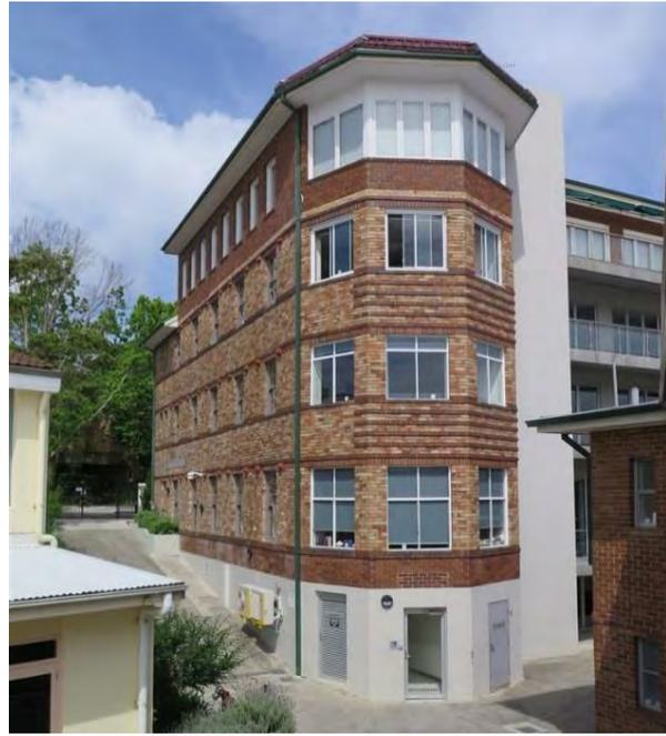
Figure 3.14 The Marian Centre, as viewed from the east. The top floor later addition can be seen. The lift shaft (later addition) is rendered and painted grey. (Source: GML, November 2016)
