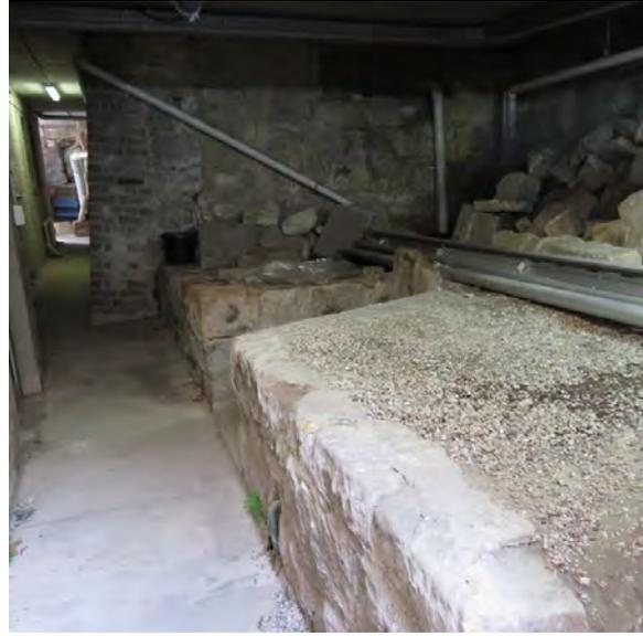
Figure 3.18 The sandstone retaining walls located below the concrete paving slab and timber deck between the Marian Centre and B-Block. (Source: GML, November 2016)
