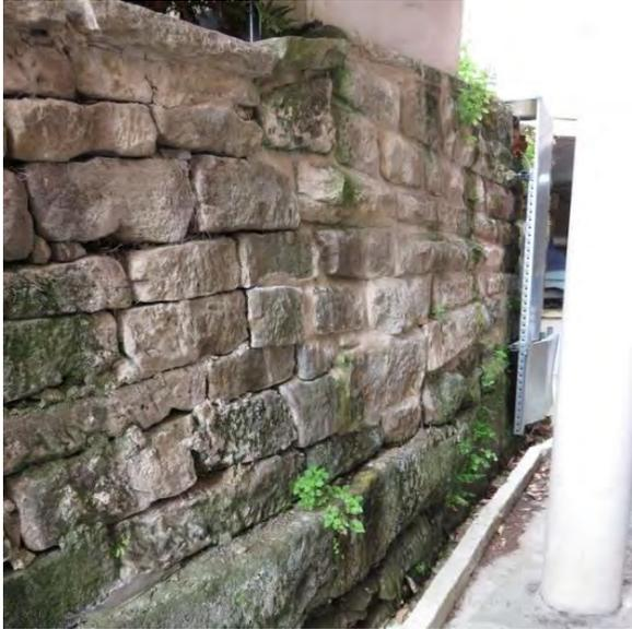
Figure 3.17 The sandstone retaining walls located between the Marian Centre and B-Block. This higher section of the retaining walls is largely intact. (Source: GML, November 2016)
