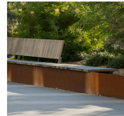
Hardwood Timber Seating on Steel Edge
