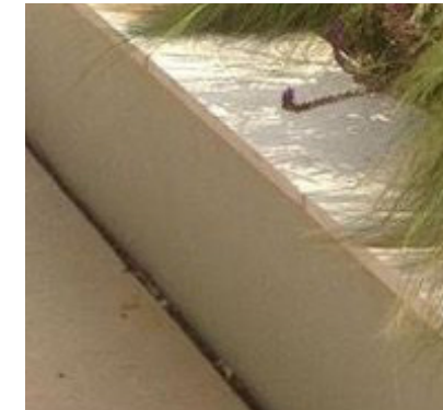
Integrally coloured and lightly exposed concrete
