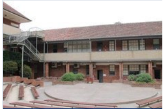
Figure 8 | Robert Vicars building and connecting walkway within the development site (Source: Applicant's EIS 2026)
