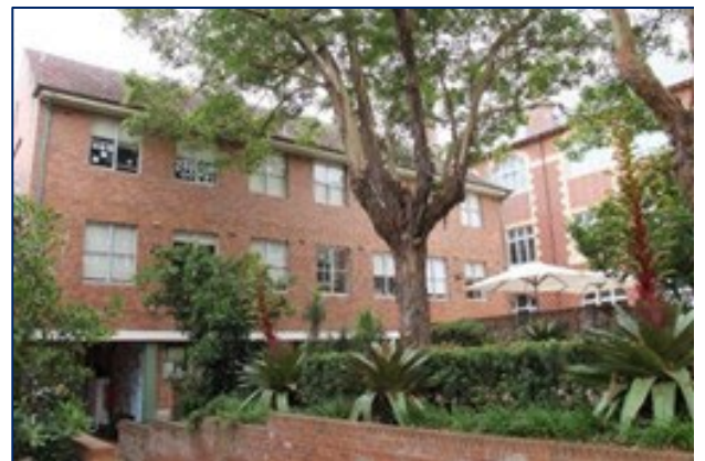
Figure 10 | John Vicars building within the development site (Source: Applicant's EIS 2026)
