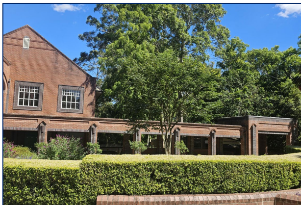
Figure 9 | Isabel McKinney Harrison building within the development site (Source: Applicant's EIS 2026)
