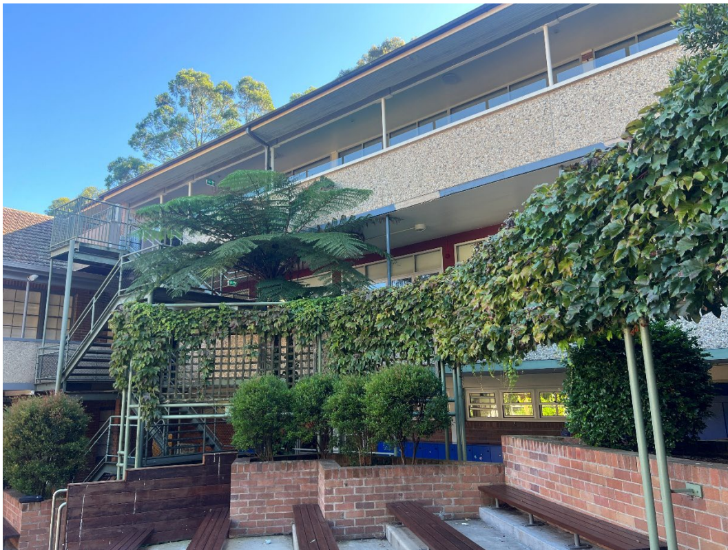
Photo 4: Showing existing Dorothy Knox Building, 14.03.2025.
