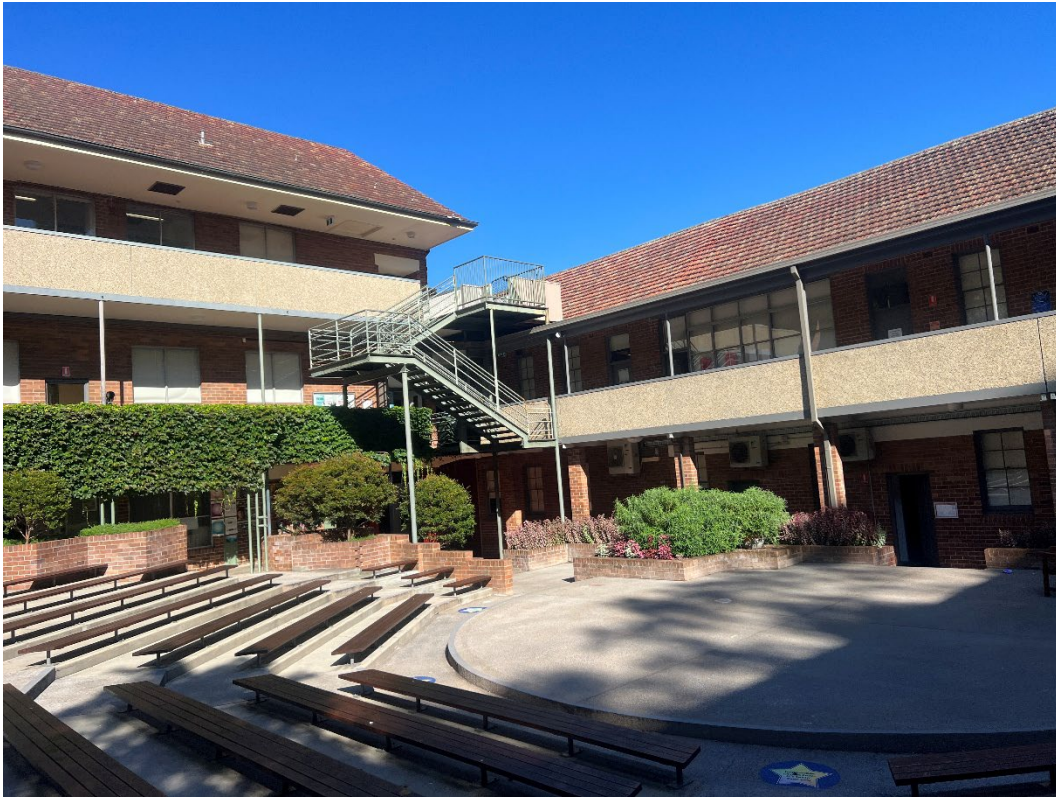
Photo 5: Showing existing Dorothy Knox Building, 14.03.2025.
