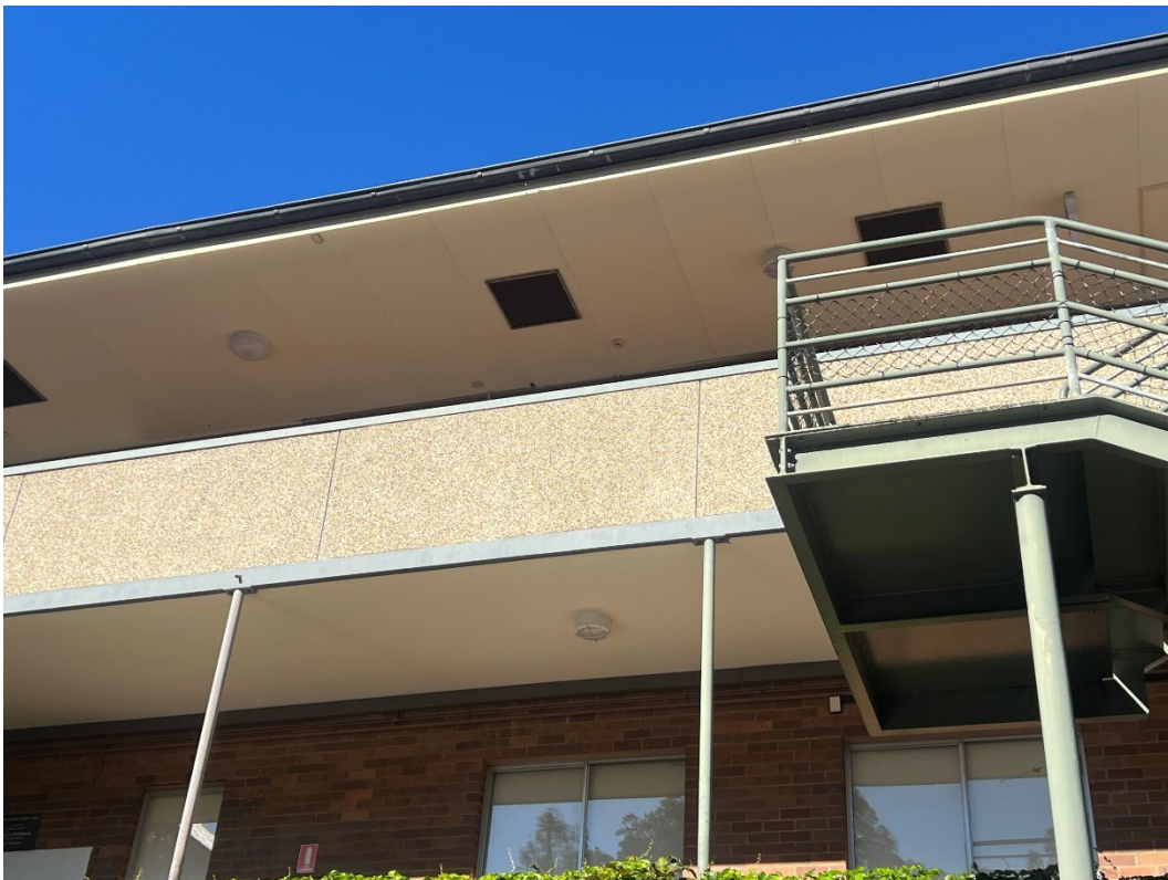
Photo 6: Showing existing Dorothy Knox Building, 14.03.2025.
