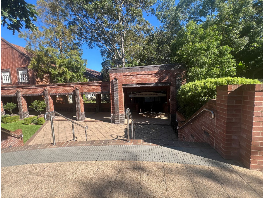
Photo 1: Showing existing Isabel McKinney Harrison Centre Building, 14.03.2025.
