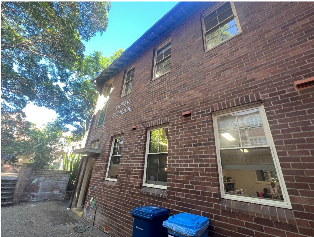
Photo 12: Showing aged building structures within the SIP and Campus Commons areas, 14.03.2025
