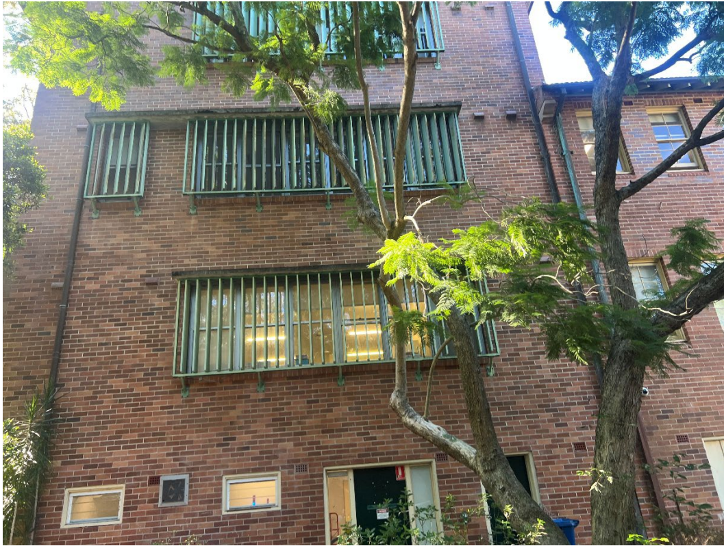
Photo 11: Showing aged building structures within the SIP and Campus Commons areas, 14.03.2025
