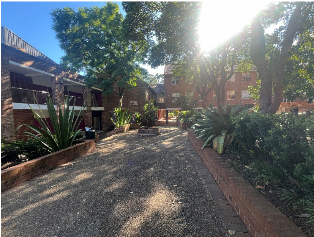
Photo 13: Showing existing aged buildings within the Campus Commons Area, 14.03.2025
