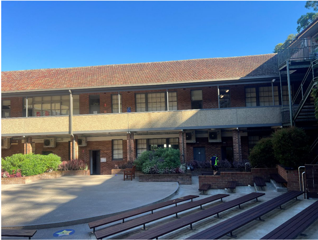
Photo 3: Showing existing Dorothy Knox Building, 14.03.2025.
