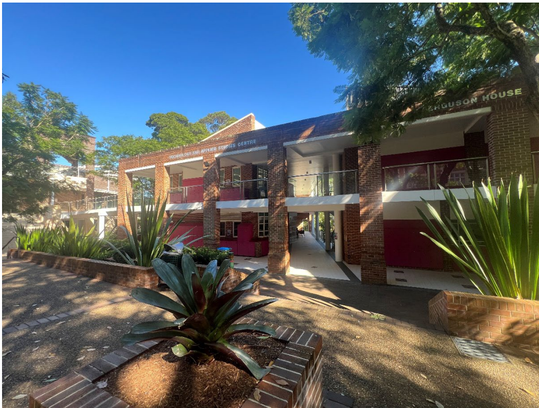
Photo 13: Showing existing Ferguson House and Applied Studies Building, 14.03.2025
