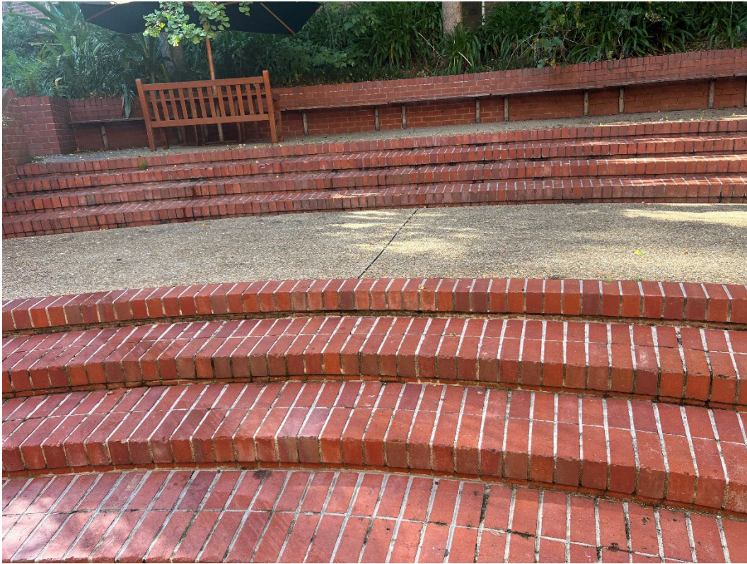
Photo 9: Showing typical hardstands throughout SIP and Campus Commons areas, 14.03.2025.
