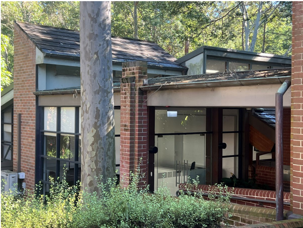
Photo 2: Showing existing Isabel McKinney Harrison Centre Building, 14.03.2025.
