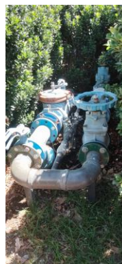
Figure 9: Existing authority water meter assembly
