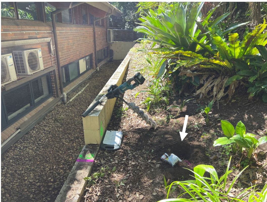
Photo 12: Showing borehole BH6 sampling location, looking north, 05.04.2025.
