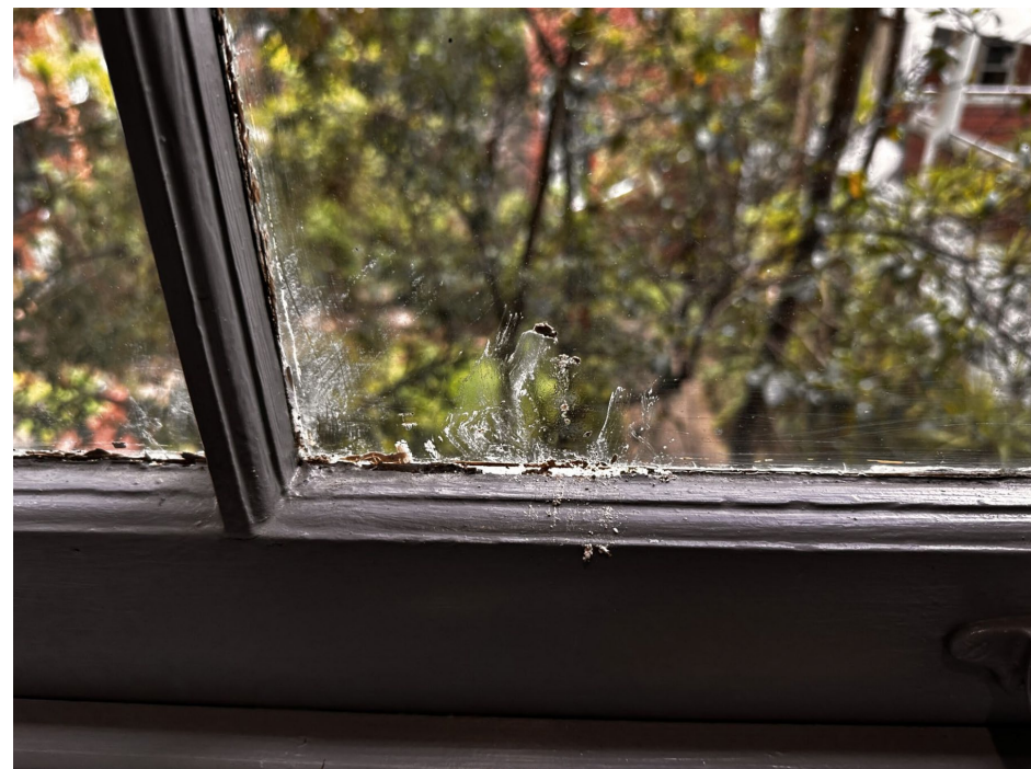
Photo 17: RVB – White mastic sample from internal window sills
