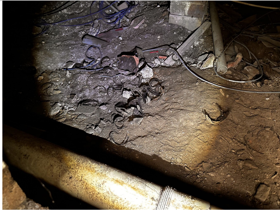
Photo 31: RVB - Subhole of manhole with black membrane spread throughout
