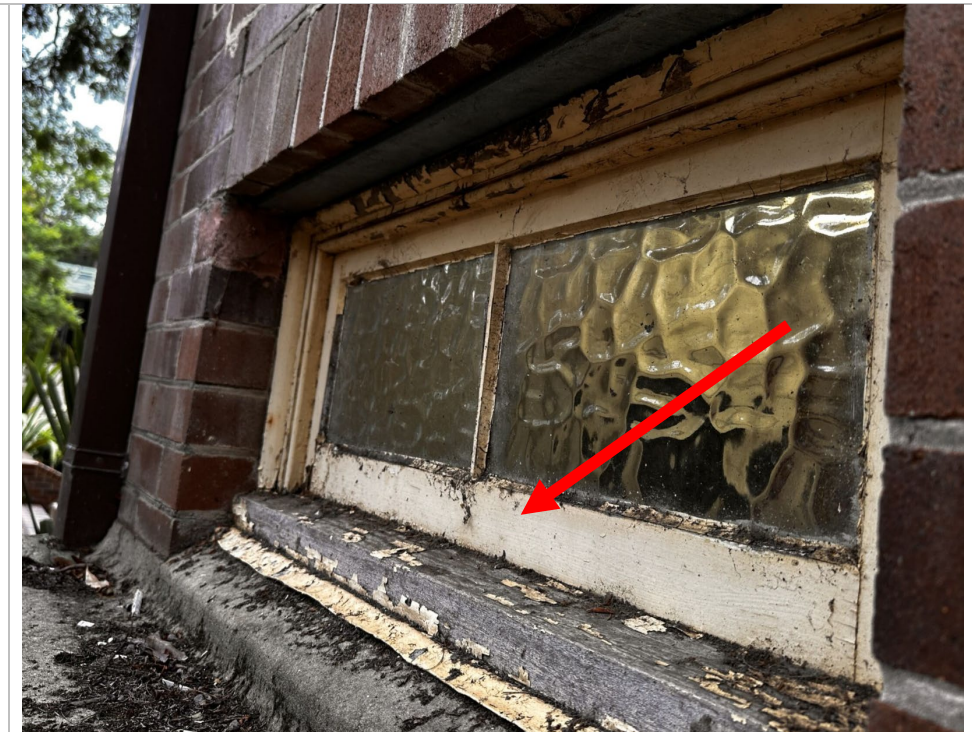
Photo 9: RVB - Sample 4 & 5 Location – Flaking paint in old cream window over door frame contains lead
