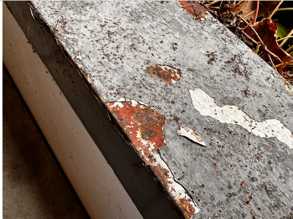
Photo 37: JVB – Grey lead paint to levels 1 and 2 rails, walls and beams
