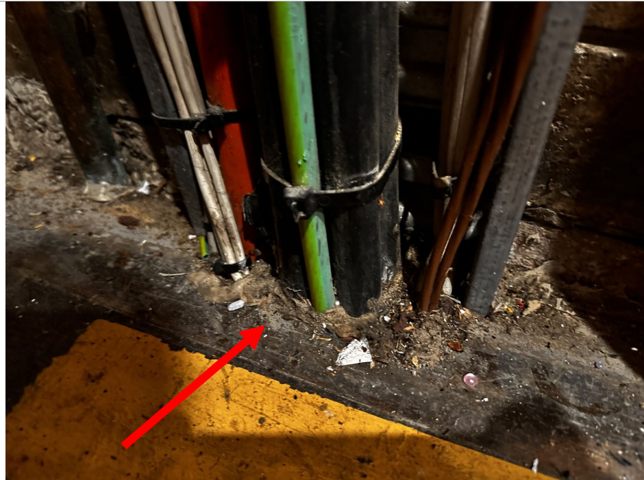
Photo 20: RVB - Old cable sheath in risers may contain asbestos.
