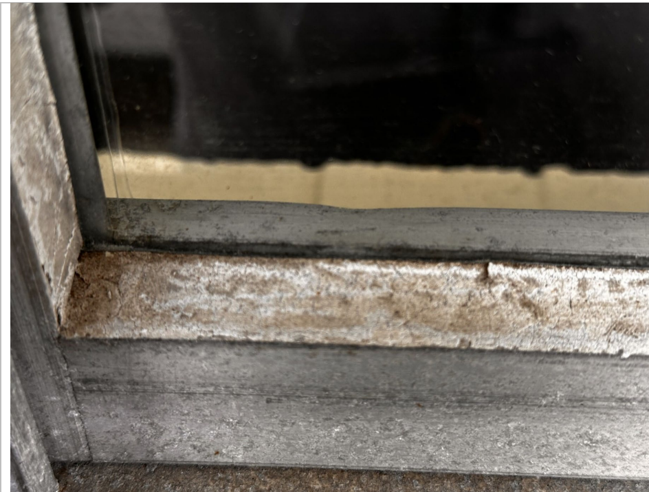
Photo 50: RVB – Mastic on window frame
