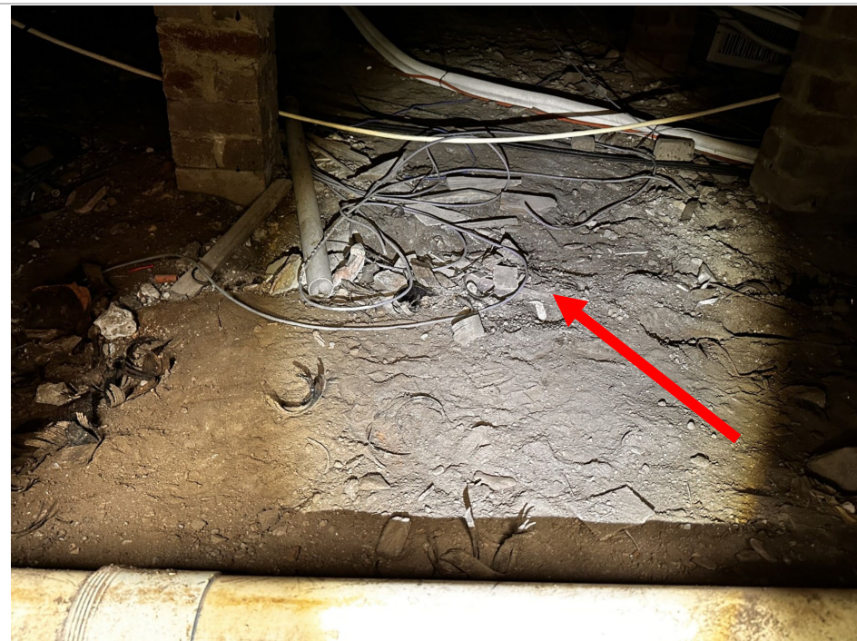
Photo 29: RVB - Subfloor of manhole; ACM fragments and debris contain asbestos.
