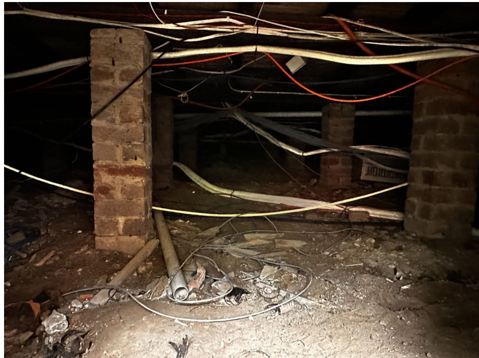
Photo 34: RVB – Internal of manhole contains asbestos debris.
