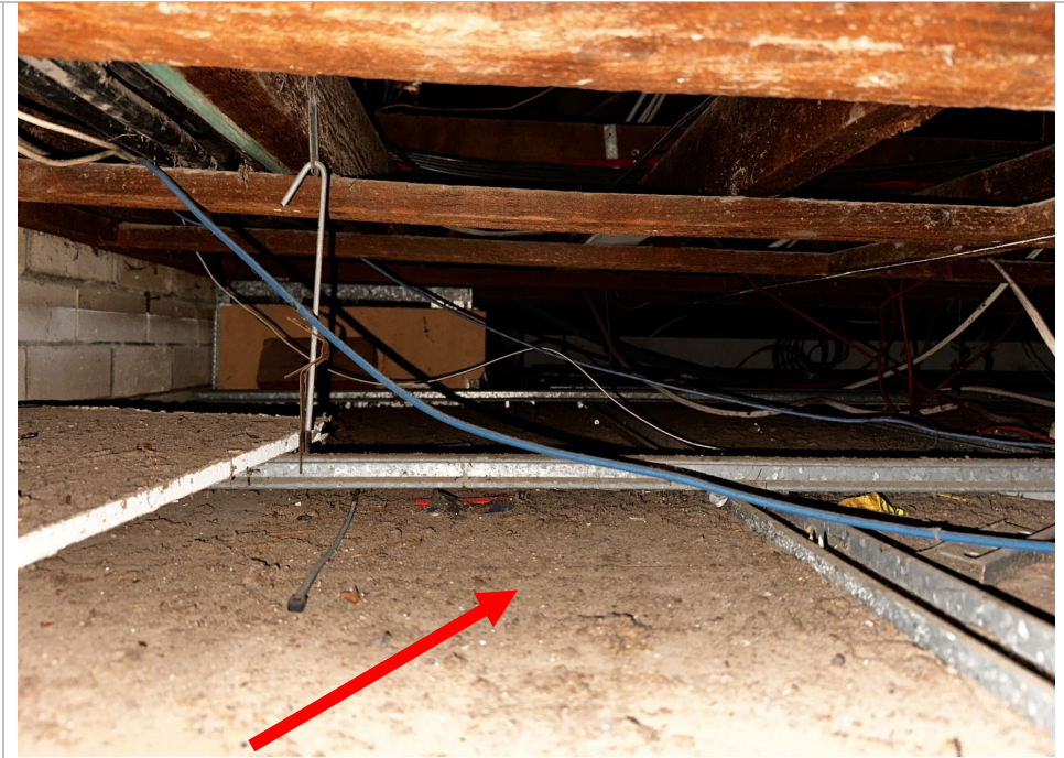
Photo 21: RVB – Asbestos ceiling Dust, location of samples 24 and 25
