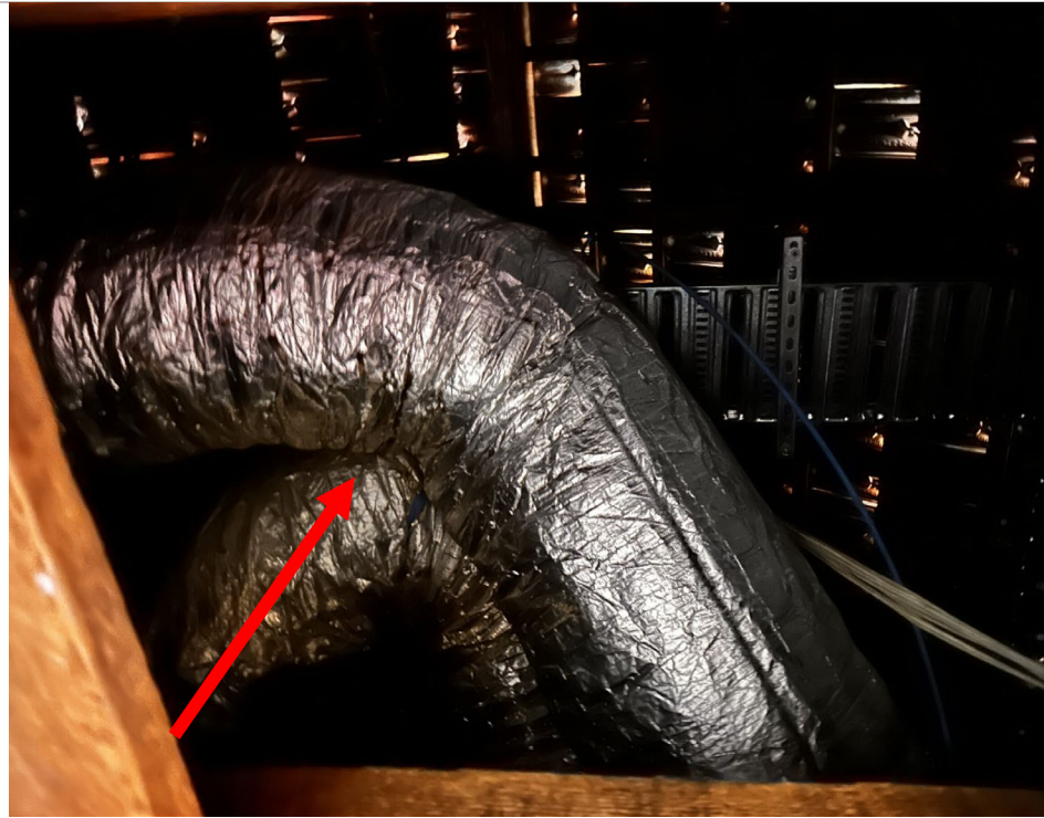
Photo 19: RVB – Synthetic mineral fibers SMF can be found in AC Ductwork
