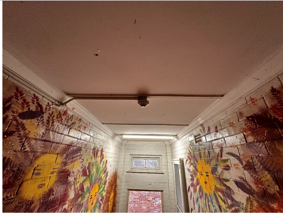
Photo 13: RVB – Ceiling above stairs contains asbestos
