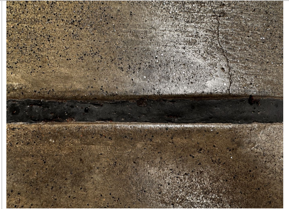
Photo 39: JVB – Expansion joint on level 1 floor
