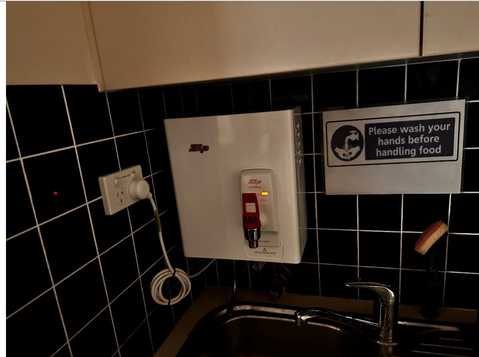
Photo 61: JVB Zip Hot Water Taps contain SMF in boilers.
