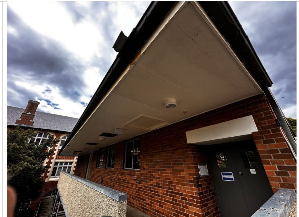
Photo 45: JVB and RVB balcony ceiling contain asbestos.
