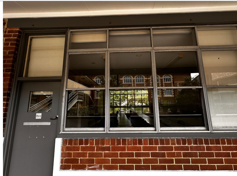
Photo 49: RVB - External steel window mastic
