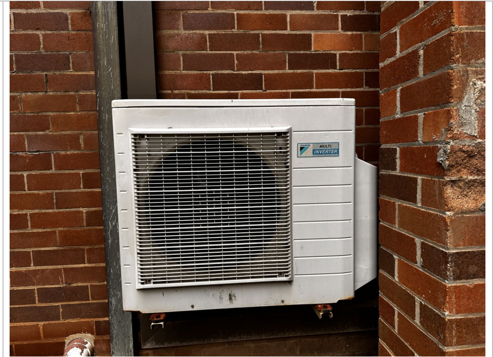
Photo 27: RVB – AC units contain SMF as well as ozone depleting substances.
