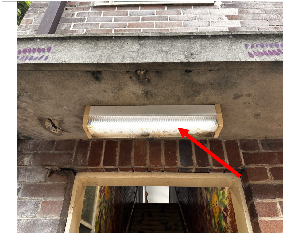
Photo 7: RVB – Mercury in floccrescent light fixtures
