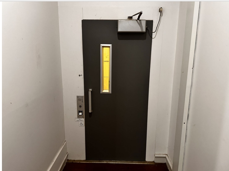
Photo 22: RVB – Dark green paint on door. Lift Door cores may contain asbestos.
