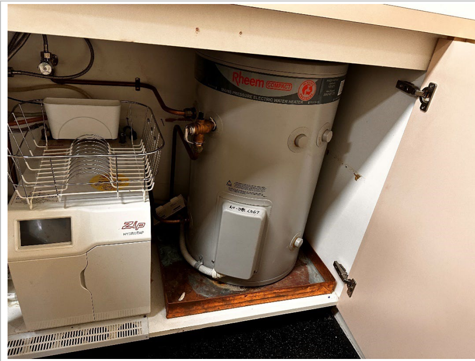
Photo 62: RVB Hot Water Heaters contain SMF.
