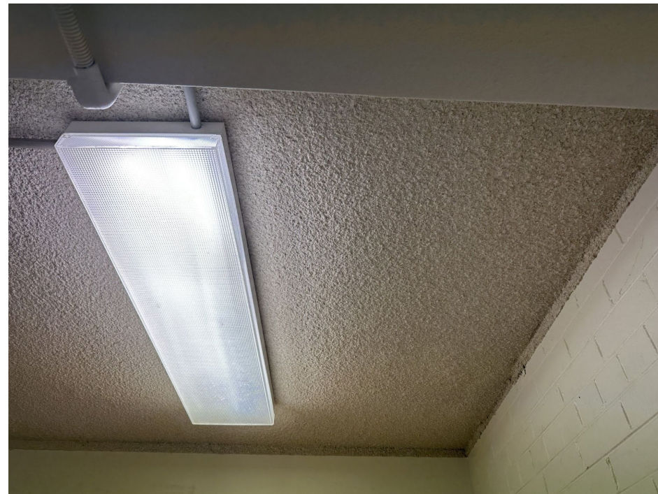
Photo 56: DKB – Archive room ceiling lights may contain mercury.
