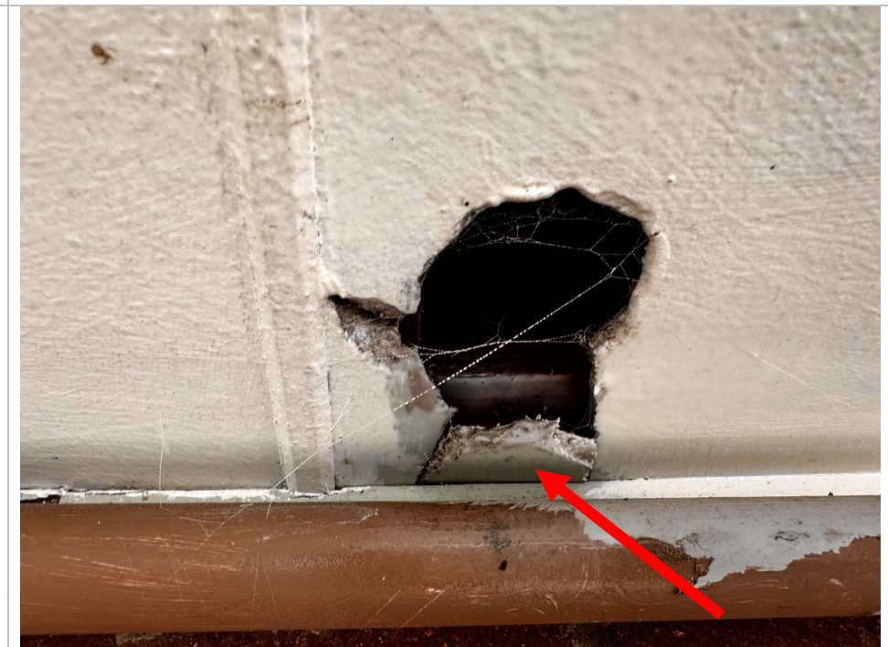
Photo 48: JVB and RVB ceiling contains asbestos and is exposed.
