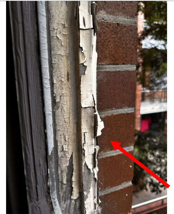
Photo 18: RVB – Deterioration on external door frame may contain lead.
