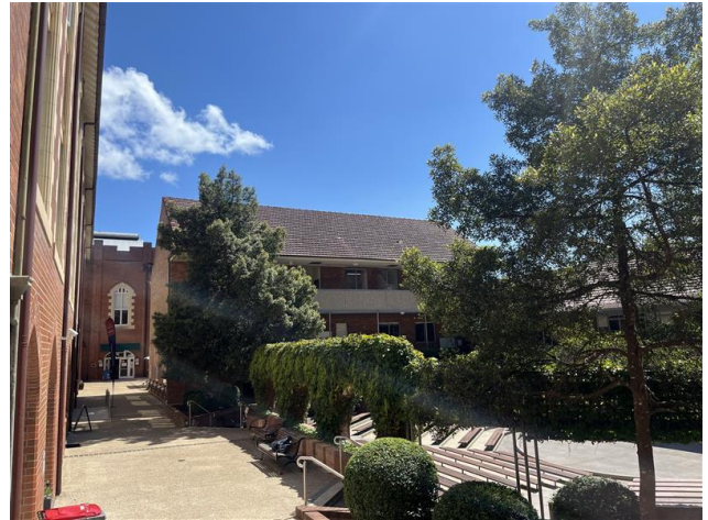
Picture 2 Robert Vicars building on the development site (to be demolished)
