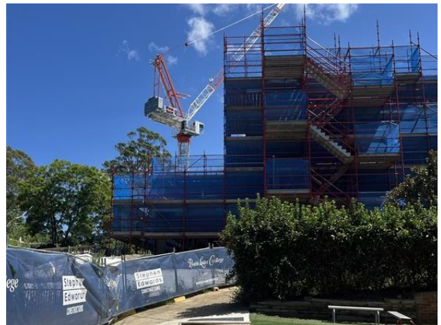
Picture 4 Grey House Precinct within the College (under construction)
