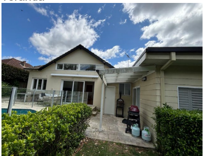
25 Roseville Avenue, Contemporary rear extension
