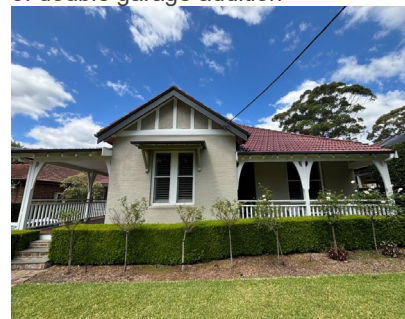
27 Roseville Avenue, Primary façade with extensive alterations
