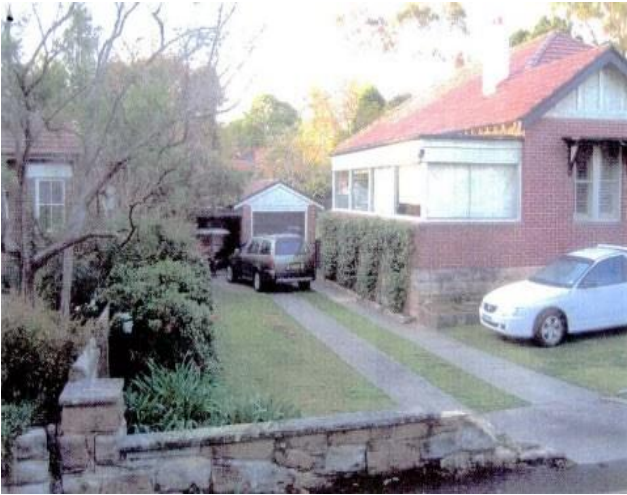
Figure 116 Photograph of dwelling in 2005 with contemporary street-facing sun room prior to reinstatement of veranda works in 2015
