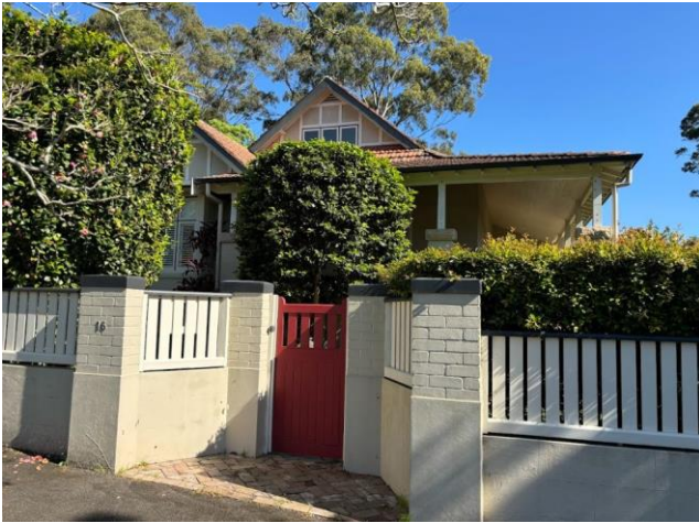
Figure 9 Primary façade view from Lord Street
