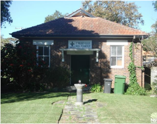
Figure 128 North Elevation of Roseville Scout Hall 2012
