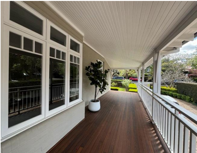
Figure 42 Contemporary side veranda, formerly covered sunroom
