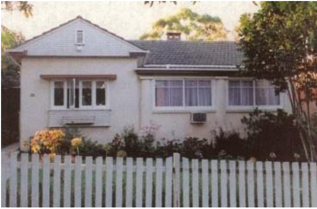
Figure 64 Primary Lord Street façade dated from 2004
