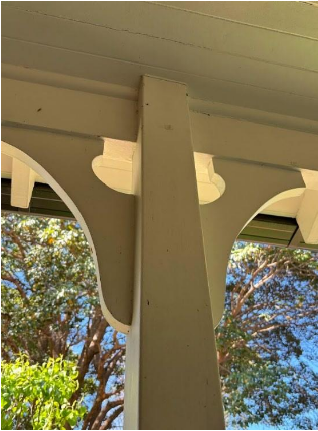
Figure 21 Timber veranda posts
