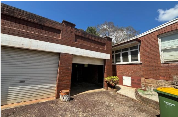
Figure 31 Front façade of double garage Source: Urbis, 10 October 2024
