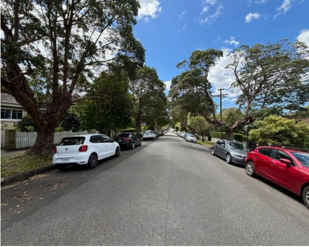
Figure 4 Looking North-East along Lord Street
