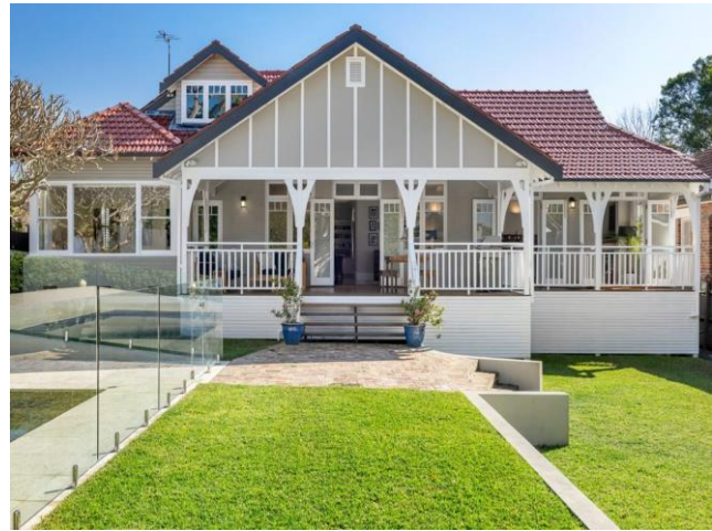
Figure 43 Rear contemporary façade of dwelling and upper attic extension dating from 2015 construction
