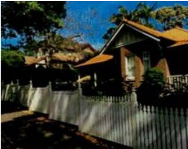
Figure 86 Photograph of primary façade of dwelling dated from 2015
