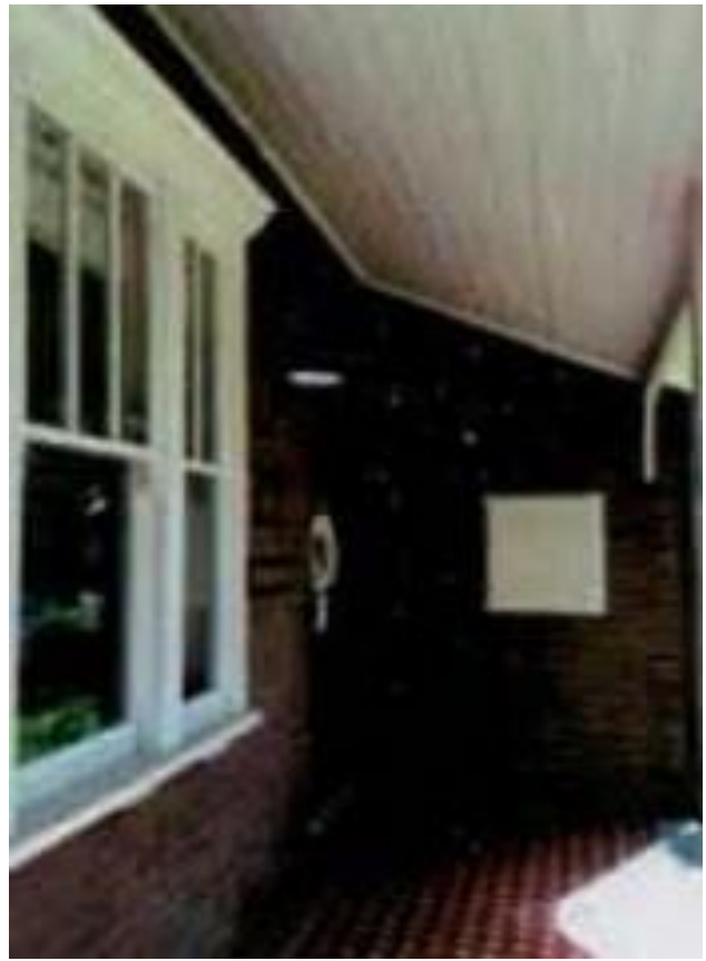
Figure 85 Photograph of front façade and veranda dated from 2015
