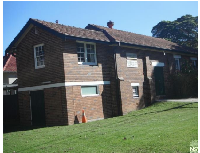
Figure 129 East Elevation of Roseville Scout Hall 2012
