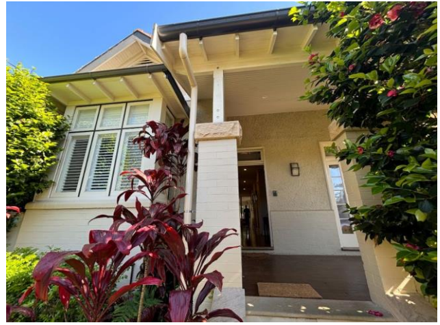
Figure 10 Close up of primary façade, original prominent gable form with contemporary veranda construction
