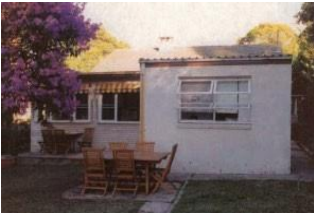
Figure 66 Rear building façade indicating contemporary rear extension dated from 2004
