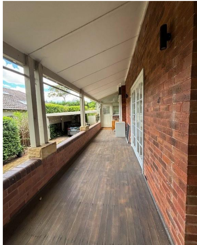
Figure 35 Contemporary veranda extension dating from 1973
