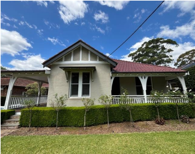
Figure 40 Primary façade of dwelling with extensive alterations to original form
