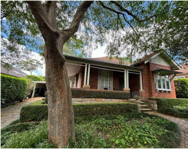
Figure 32 Dwelling with adjacent car port on the left-hand side
