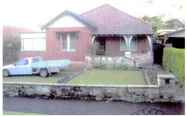
Figure 119 Photograph of front of dwelling in 2005 indicating former front veranda construction
