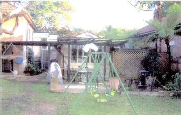
Figure 118 Photograph of rear of dwelling in 2005 indicating former 1980s covered extension and garage
