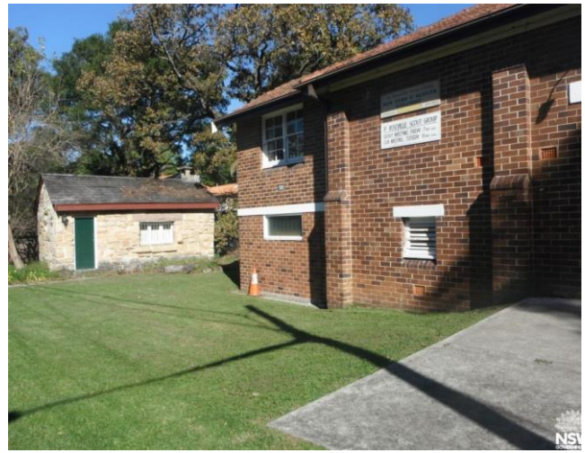
Figure 131 Side elevation and stone cottage 2012
