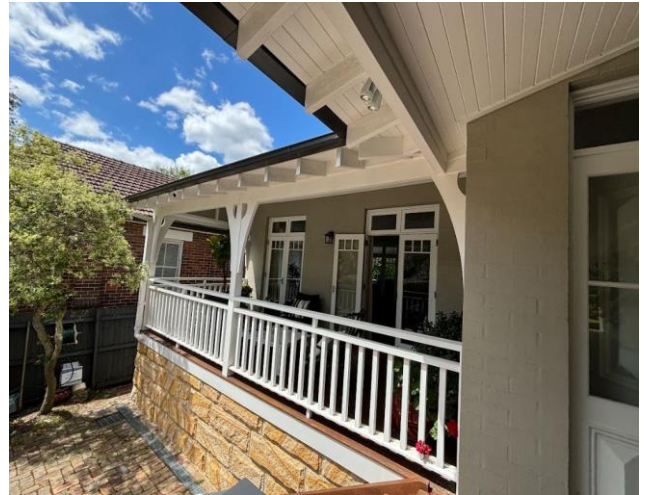
Figure 41 Set-back veranda on street-fronting façade dating from 2015 extension
