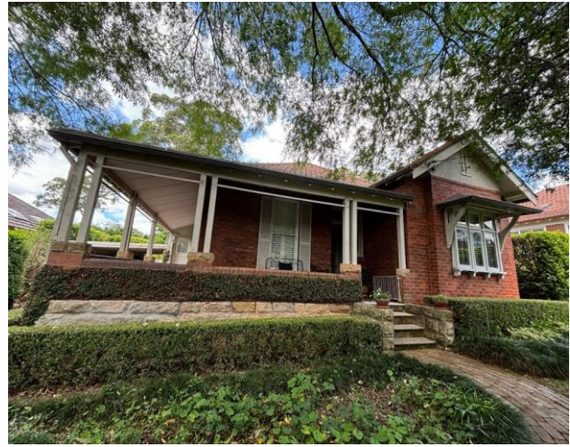
Figure 33 Primary façade of dwelling with contemporary veranda extension on left-hand side
