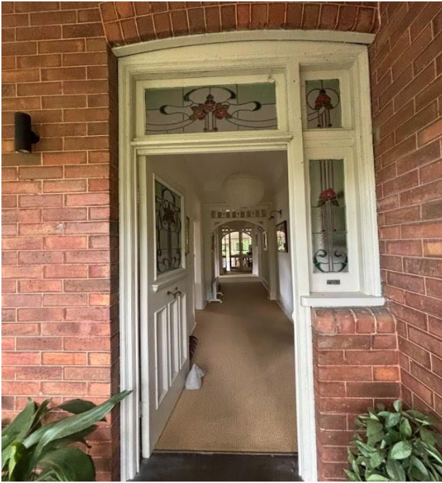
Figure 36 Reconstructed lead light front entry door Source: Urbis, 10 October 2024
