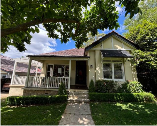
Figure 38 Plain street facing façade of subject dwelling bounded by low-rise shrubbery
