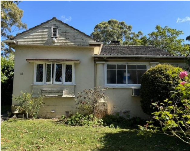
Figure 13 Primary façade view from Lord Street
