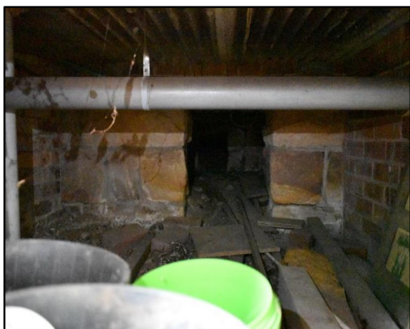
Figure 49: 23 Roseville Ave, basement.
