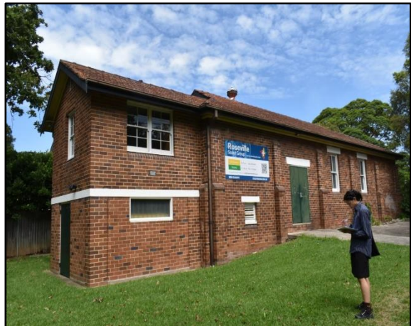
Figure 38: Roseville Scout Hall, facing west.
