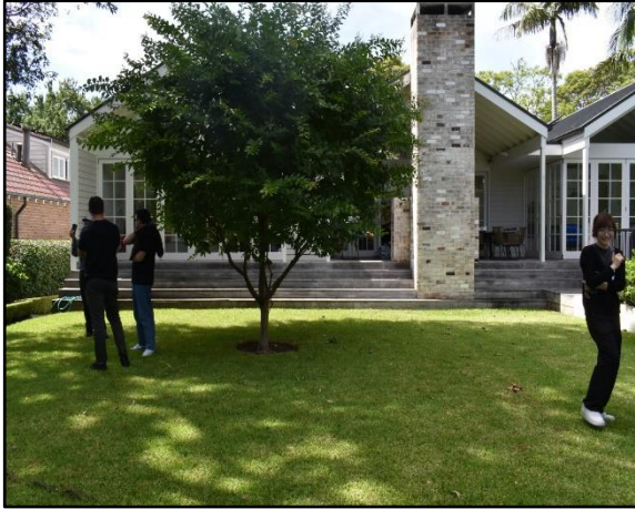
Figure 33: 22 Lord St, house from backyard.
