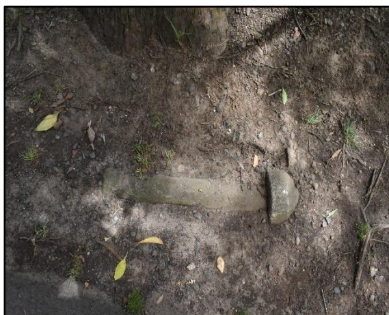
Figure 50: 23 Roseville Ave, concrete pipe.
