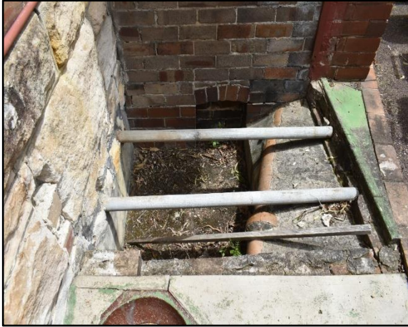
Figure 51: 21 Roseville Ave, house foundations and pipe.
