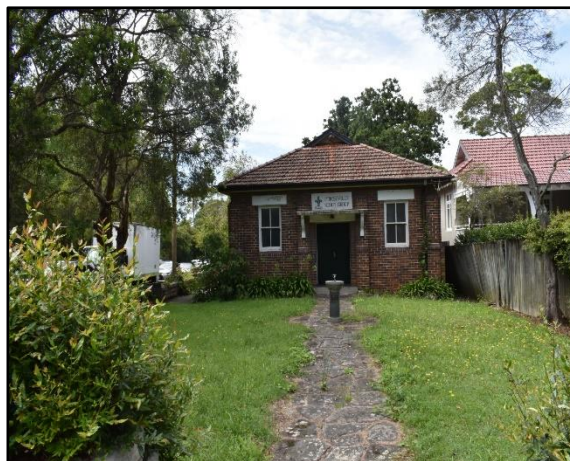
Figure 40: Roseville Scouts Hall facing southwest.
