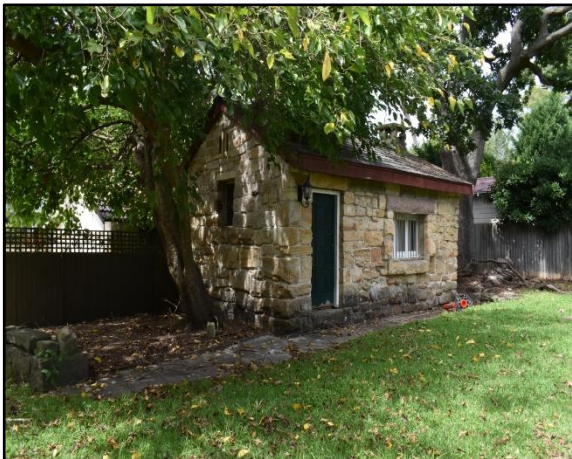
Figure 37: Small structure associated with the Roseville Scout Hall.
