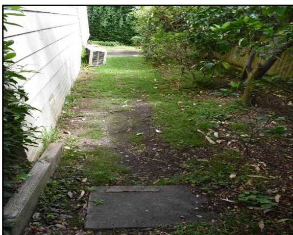
Figure 43: 25 Roseville Ave, side backyard.
