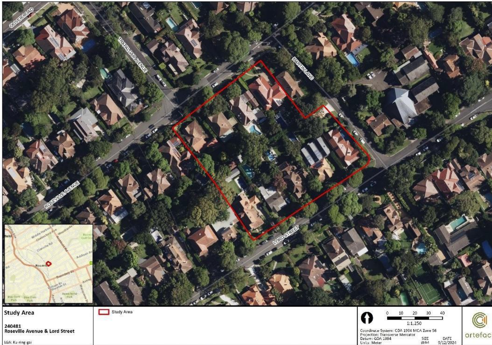
Figure 4: Aerial view of the site bounded by Lord Street and Roseville Avenue (source: Artefact)
