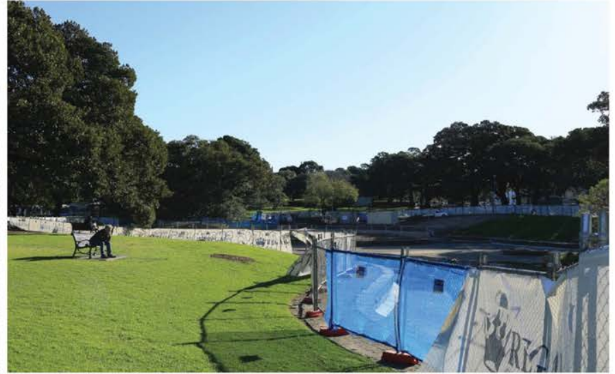
Location 5; View west towards the location of the Quad and Great Hall.
