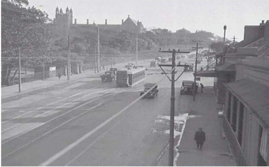
Location 1; View west along Parramatta Road from near Derwent Lane circa 1930.
