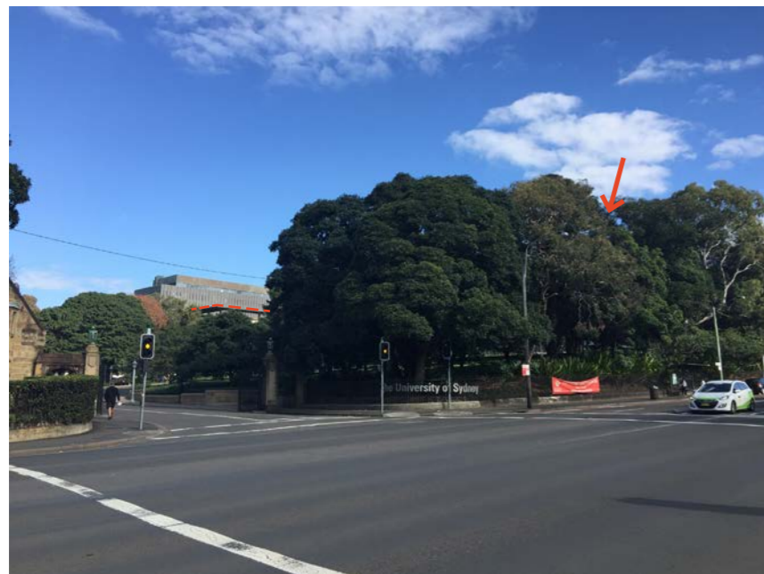
View from Parramatta Road & University Avenue, 2016
