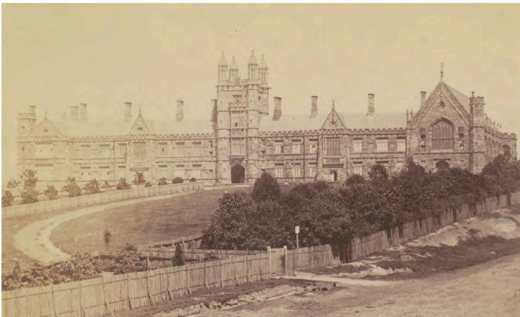
Figure 7. 1869 View from Parramatta Road
