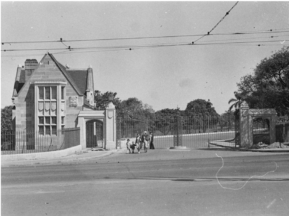
Figure 19. Parramatta Road Gates and Lodge 1940
