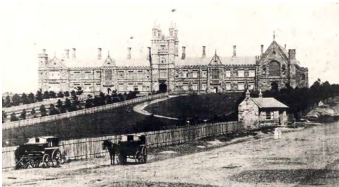
Figure 4.4 University Building viewed from Parramatta Road (undated, between 1865 - 1885)
