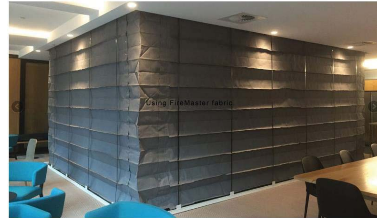
Figure 31 Concertina fire curtain: picture taken from "Greene" fire curtains
