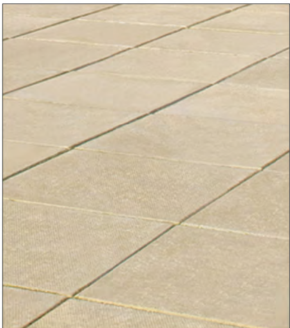
PRECAST CONCRETE PAVING
