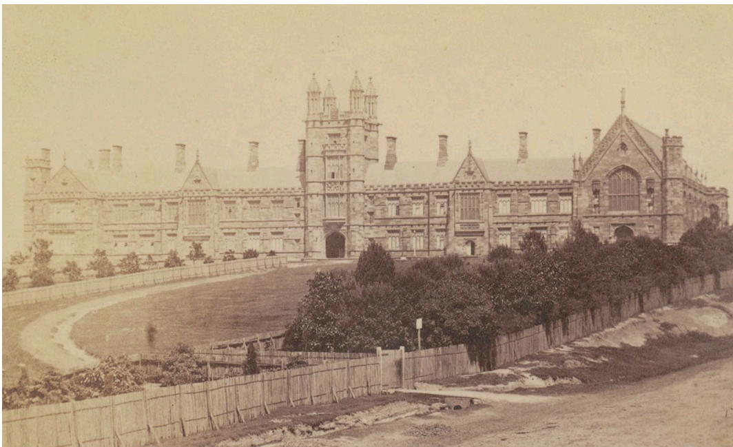
Figure 7. 1869 View from Parramatta Road
