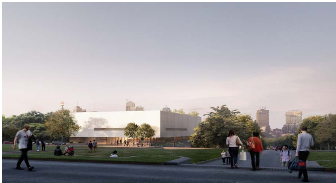
Figure 19: View of the Museum from the Quadrangle Clocktower entrance
