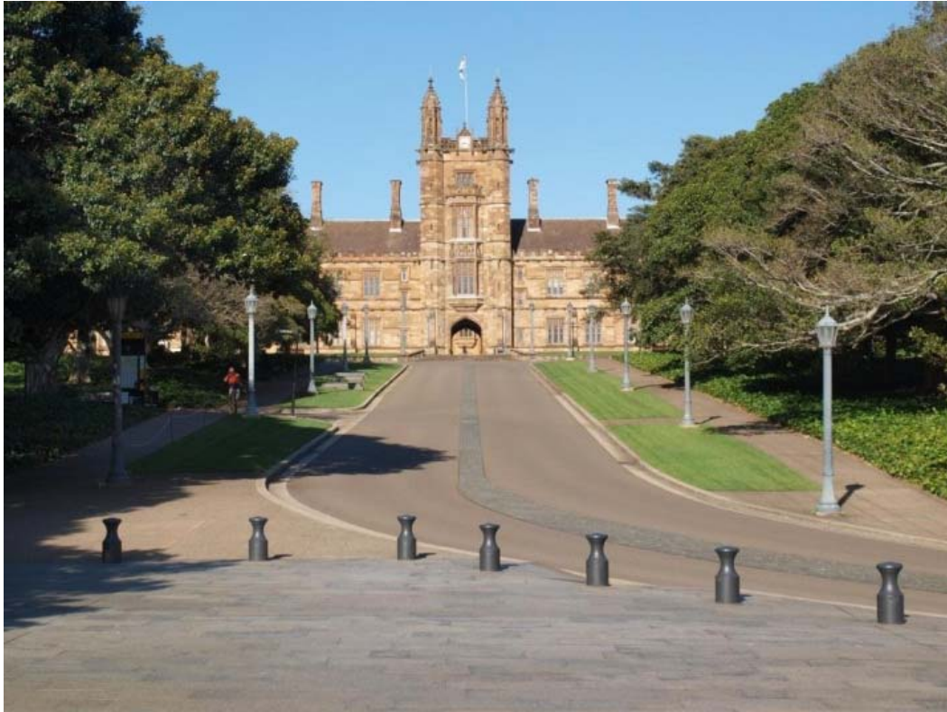
Photo 6: View to Great Hall looking west from University Avenue (CCWM site to right of picture)
