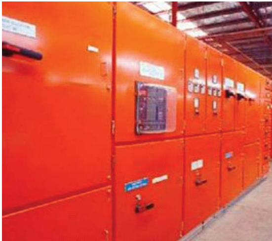
Figure 16 MSB and Temporary Generator Connection Facilities
