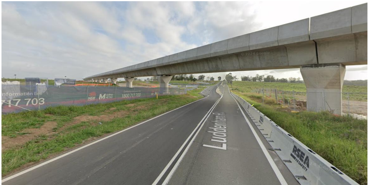
Figure 8 – Existing Viaduct Street View
