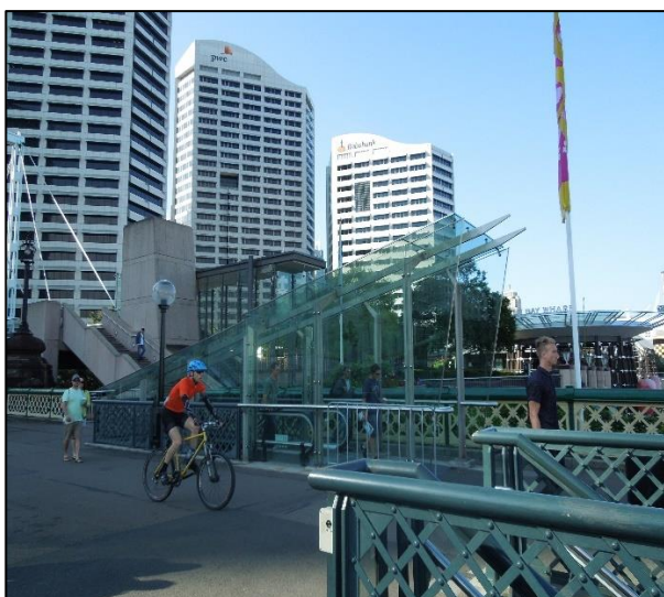
FIGURE 47: THE PROVISION OF NUMEROUS TYPES OF ACCESS POINTS HAVE HAD A PHYSICAL AND VISUAL IMPACT ON THE CITY END OF THE BRIDGE.
