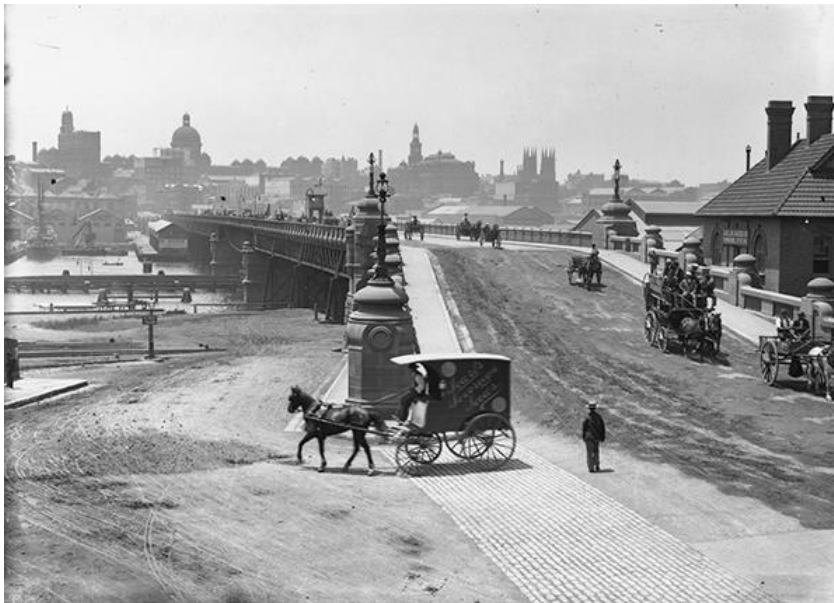
Figure 14. Pyrmont Bridge c1907 seen from its western approach. On the right is the 1902 Darling Harbour Railway Yard Goods Office (Forwarding Station) fronting the bridge. The 1891 and 1902 Outward Goods Sheds are in the background. The railway line continues under the bridge to Pyrmont and Darling Island. Powerhouse Museum, Tyrrell Collection 14-1, http://from.ph/459785
