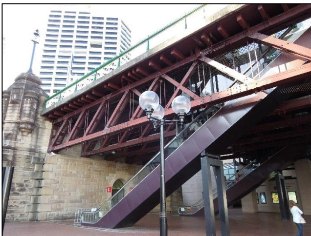
FIGURE 45: AT THE CITY END OF THE BRIDGE (EASTERN END) THE PROVISION OF ESCALATOR ACCESS HAS HAD A SUBSTANTIAL VISUAL AND PHYSICAL IMPACT ON THE QUALITIES OF THE BRIDGE.
