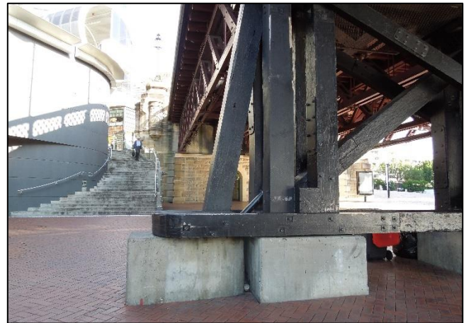
FIGURE 38: THE STAIR HAS BEEN CONSTRUCTED TO ABUT THE BRIDGE.
