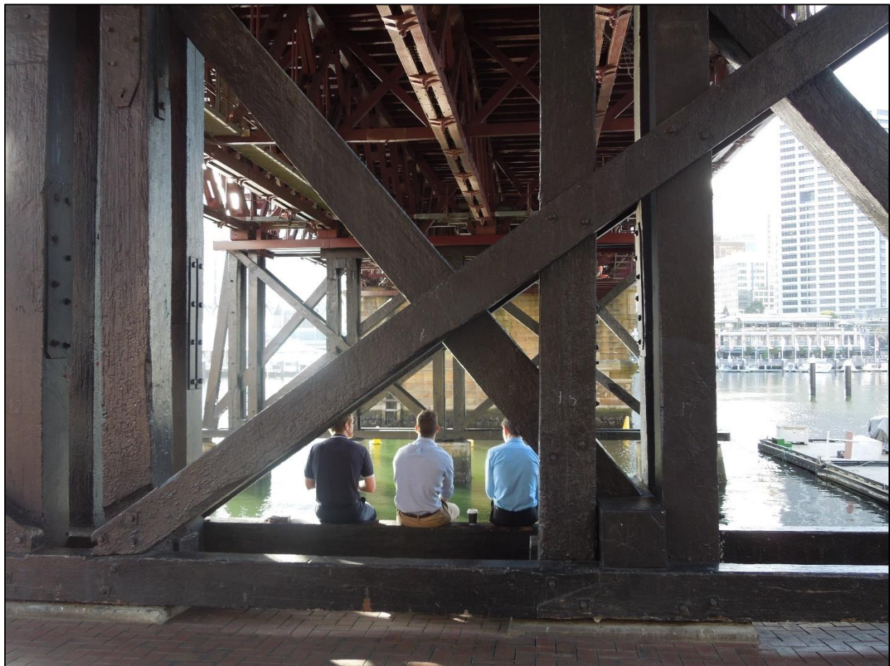
FIGURE 51: CITY WORKERS FIND A SPOT UNDERNEATH THE BRIDGE TO HAVE A BREAK AND ENJOY THE VIEWS. THIS TYPE OF ACTIVITY IS STRONGLY ENCOURAGED IN THE PUBLIC DOMAIN DESIGN AND CONCEPT FOR THE TERRACED STEPS AROUND THE TOWER PODIUM.
