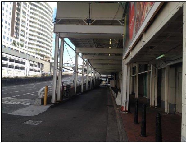
FIGURE 16: LOADING DOCK ENTRANCE ON WESTERN SIDE OF HARBOURSIDE. DARLING DRIVE RISES ON THE LEFT HAND SIDE.
