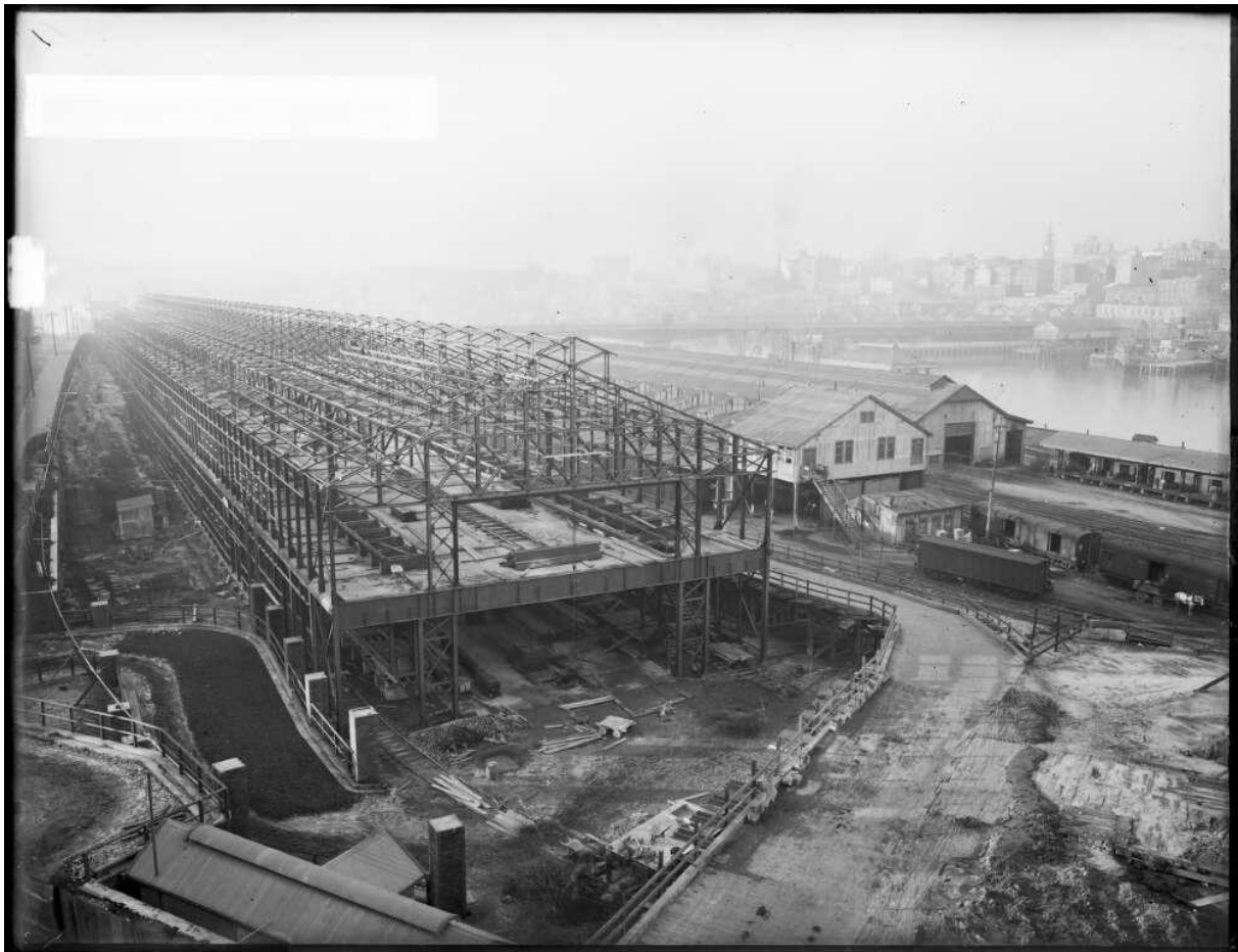
Figure 15. Construction of the Double Tier Goods Shed c1916–22. The Outward Goods Shed C & D (1891), Outward Goods Shed A & B (1902) and the covered platform are in the background. National Library of Australia, PIC P860/326, http://nla.gov.au/nla.obj-142764019
