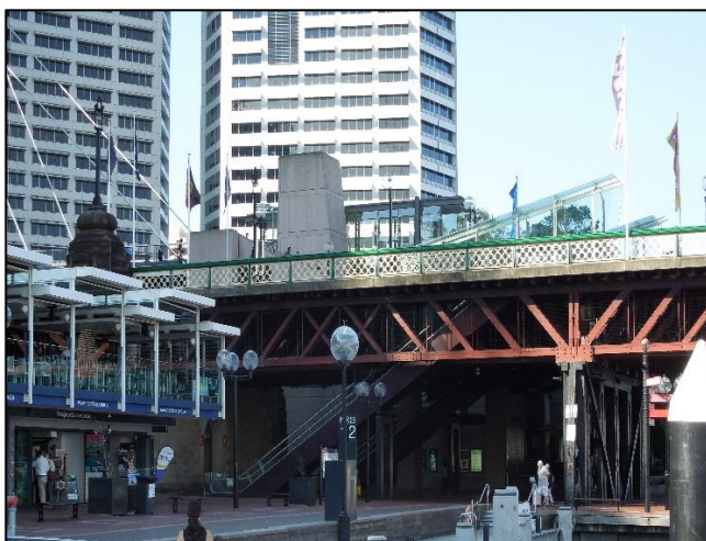
FIGURE 49: THE IMPACT OF THE STAIRS, ESCALATORS AND LIFTS ARE READILY VISIBLE FROM KEY AREAS OF THE PROMENADE (EASTERN END).
