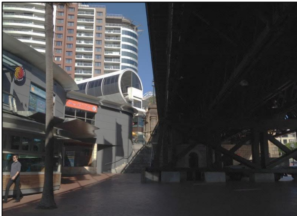
FIGURE 12: INTERFACE BETWEEN HARBOURSIDE (LEFT) AND PYRMONT BRIDGE (RIGHT), VIEW FACING WEST. THE FORMER MONORAIL STATION IS VISIBLE IN THE CENTRE OF THE IMAGE.
