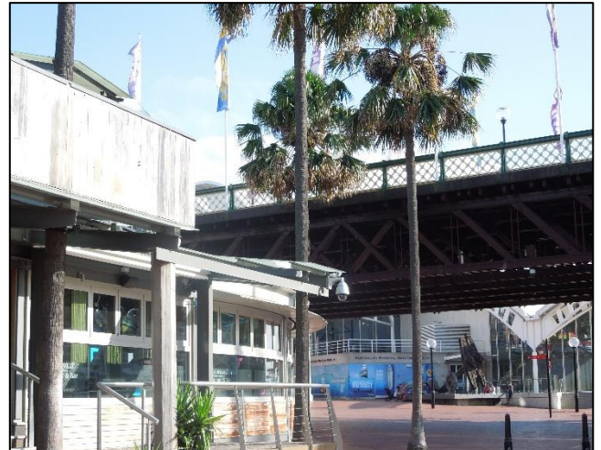
FIGURE 36: THE SITING OF THE EXISTING SHOPPING COMPLEX TOO CLOSE TO THE BRIDGE COMPLETELY OBSCURES THE SIGNIFICANT BRIDGE APPROACHES.
