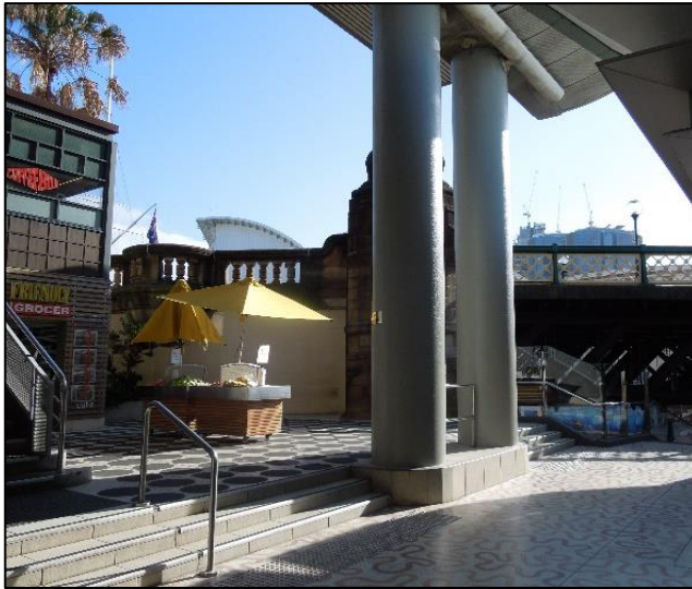
FIGURE 31: BUILDING COLUMNS AND POORLY LOCATED SHOPS HAVE A MAJOR IMPACT ON THE VISIBILITY OF THE BRIDGE.
