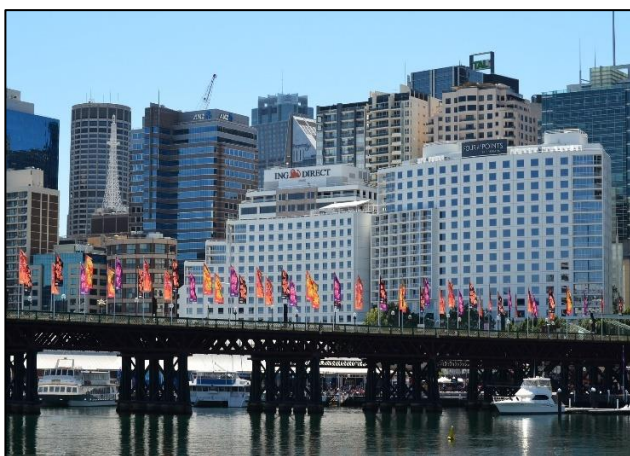
FIGURE 24: VIEW OF PYRMONT BRIDGE LOOKING NORTH- EAST TOWARDS THE CITY FROM DARLING HARBOUR. SOURCE: WALLPAPERRS.COM
