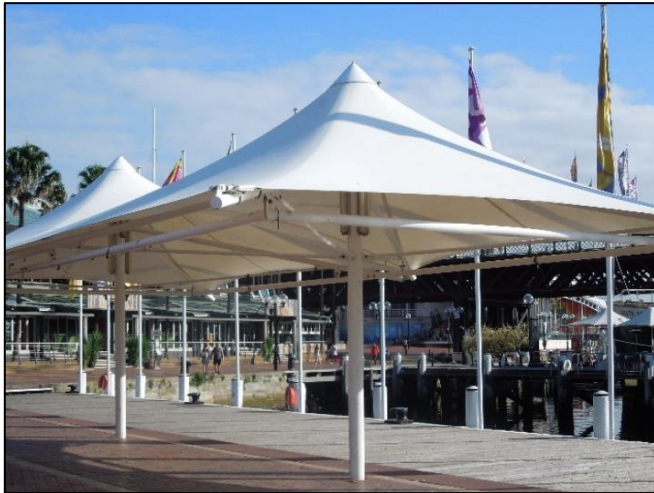
FIGURE 35: THE FIXED UMBRELLAS, WHILST PROVIDING MUCH NEEDED SHADE, OBSTRUCT VIEWS TO THE BRIDGE AND BRIDGE APPROACHES
