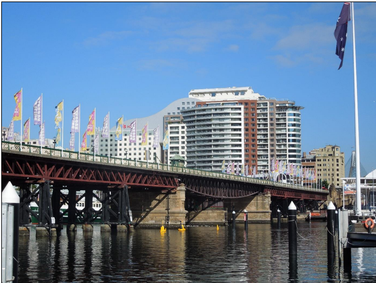
FIGURE 19: PYMONT BRIDGE LOOKING TOWARDS DARLING HARBOUR (WESTERN SIDE)
