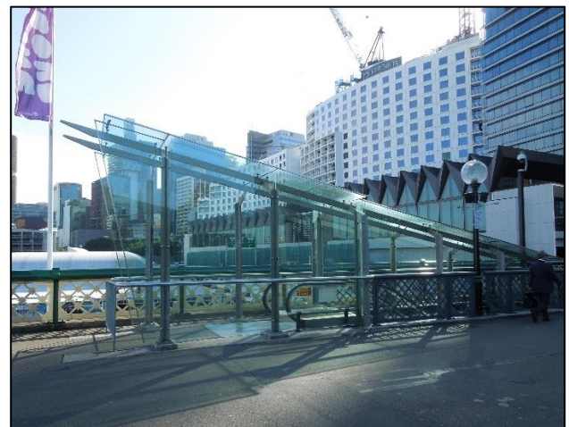
FIGURE 46: THE COVERED ESCALATORS (EASTERN END) ARE HIGHLY VISIBLE AND HAVE REQUIRED THE REMOVAL OF DECK FABRIC.
