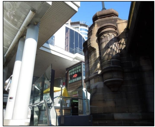
FIGURE 30: LACK OF SEPARATION BETWEEN EXISTING BUILDINGS AND SIGNIFICANT HERITAGE FABRIC OF THE BRIDGE.
