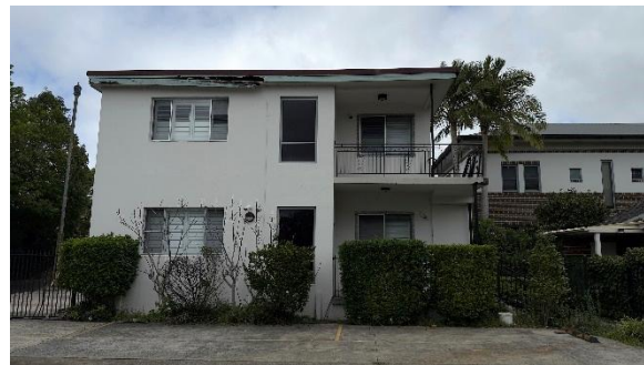
Figure 15. 27 Tryon Road rear wing addition, looking west.
