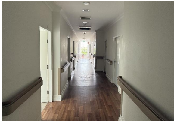
Figure 21. Internal view of typical corridor leading to patient ward rooms.
