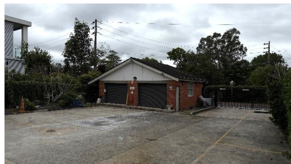
Figure 17. View of rear garage outbuilding, looking southeast.
