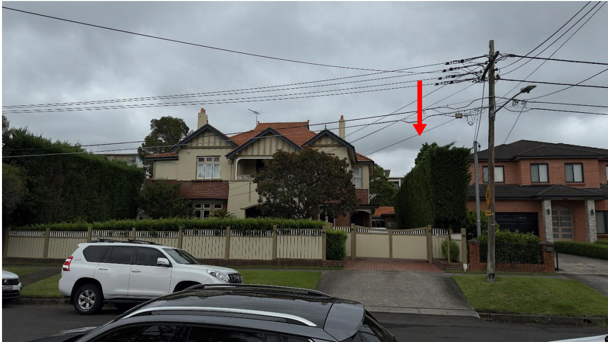
Figure 42. View 3 - from Russell Avenue, looking northwest. The approximate location of the subject site is indicated by the red arrow.
