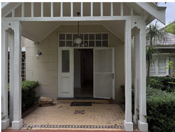
Figure 30. View of front (northern) entrance.
