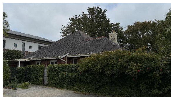
Figure 27. 29 Tryon Road rear (southern) elevation.
