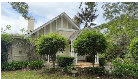
Figure 26. 29 Tryon Road northern elevation.
