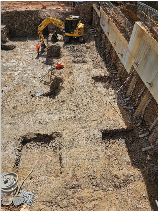
Photo 1- Basement in shale at up to 8m depth
