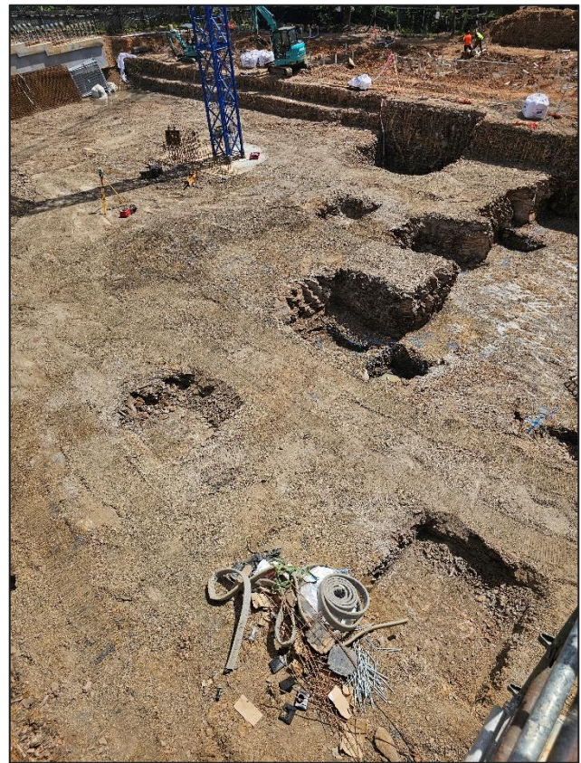
Photo 2 – Footing excavation in process.
