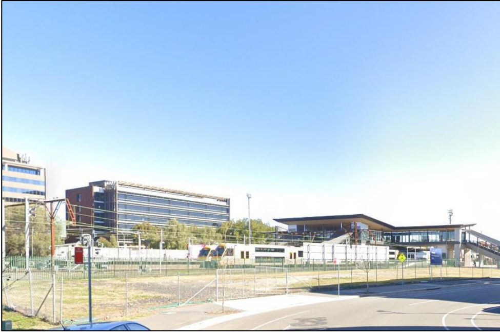
Figure 4: Looking towards the site from the east on Lord Sheffield Circuit. Provided by the client
