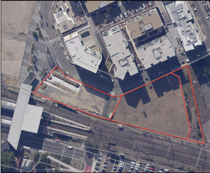
Figure 2: Aerial photograph of Nos. 160, 162 and 172 Lord Sheffield Circuit. The site is outlined in red. SIX Maps 2025
