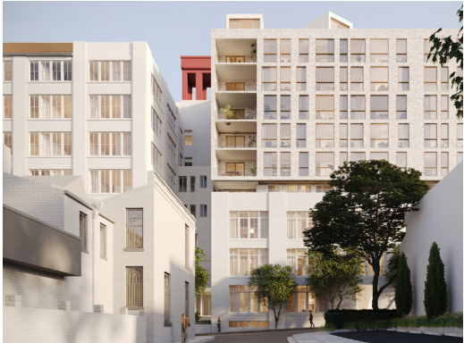
② Removal of later elements to expose original heritage fabric and introduce courtyard between South and Central building.
