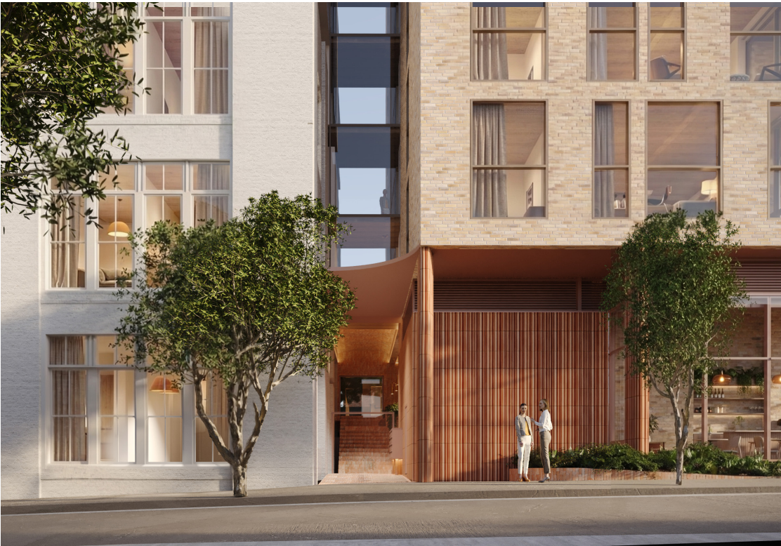
A. North Building Entry
