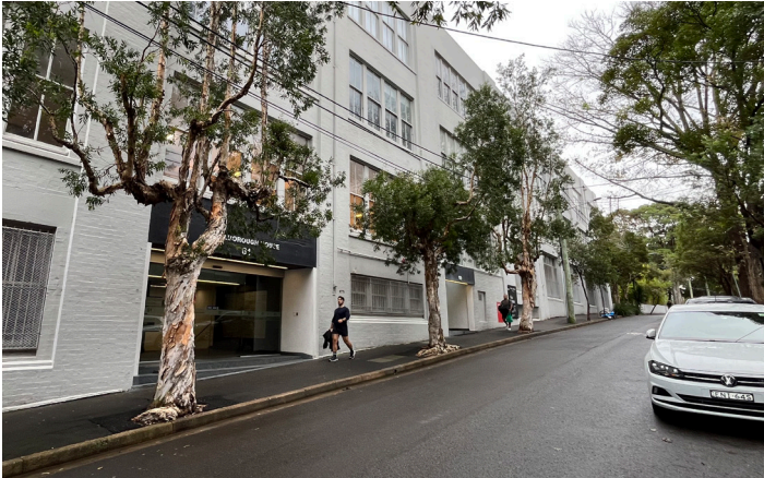
Marlborough St - 6m level different
