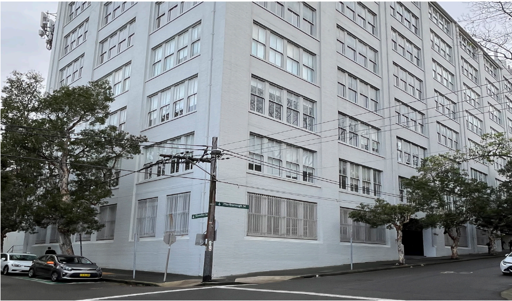
Existing - Corner View
