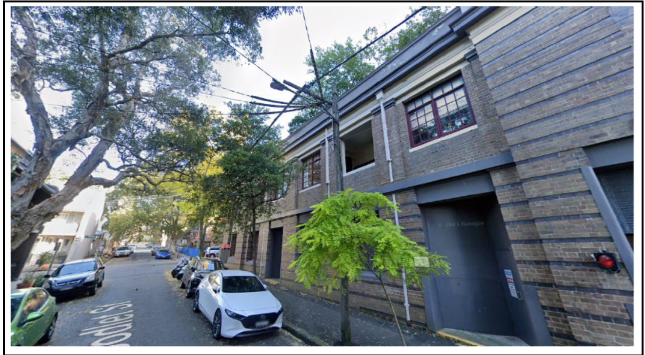
Figure 7 – LV Overhead conductor in the vicinity of the Site (Source: Google)
