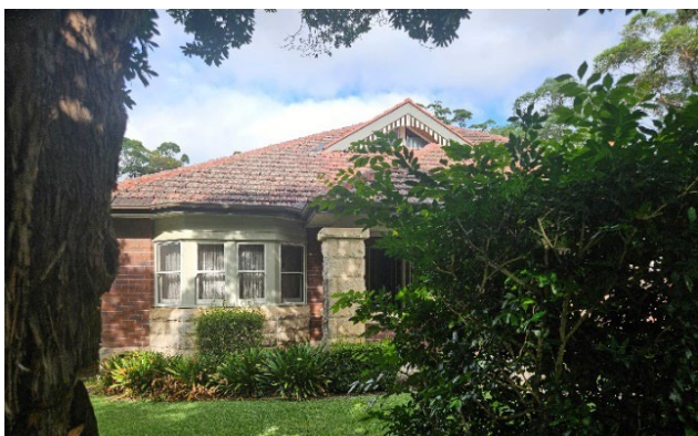
Figure 22 View of front façade.
