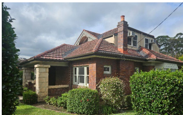
Figure 23 Front façade viewed from southwest.
