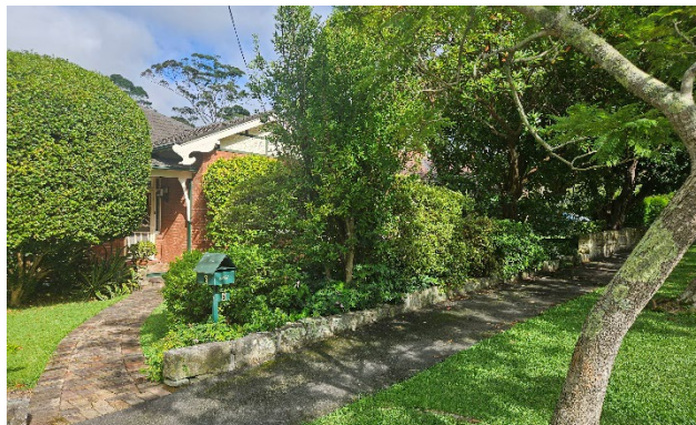
Figure 19 View of front façade – which is obscured by vegetation
