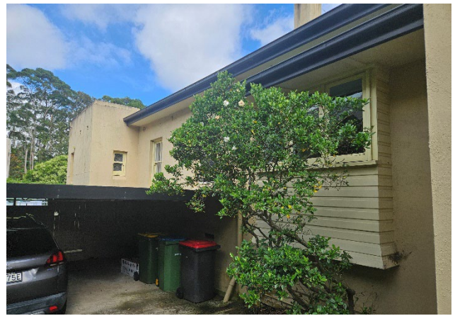
Figure 17 View of the southern façade.
