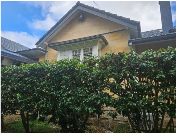
Figure 10 Front façade, showing alterations, with contemporary tiling as a decorative feature of the façade.
