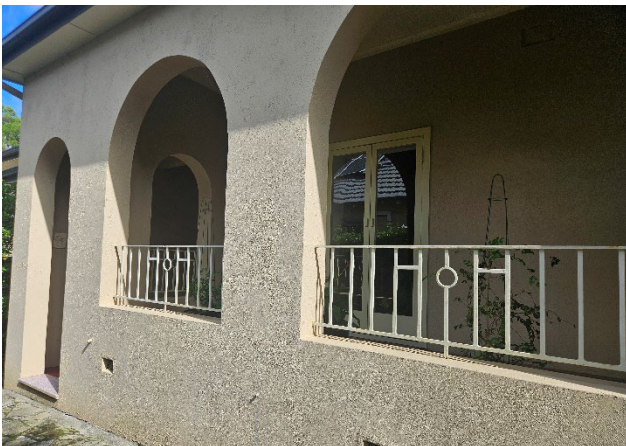
Figure 16 View of the southern façade.
