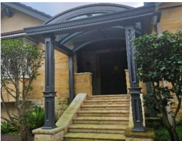
Figure 12 Front façade, showing alterations, with contemporary tiling as a decorative feature of the façade and stone staircase entry.
