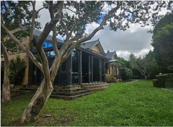
Figure 8 View looking northeast to the front façade, showing alterations to the dwelling in the foreground.
