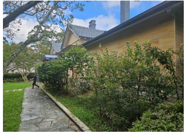
Figure 9 View looking west along front façade.
