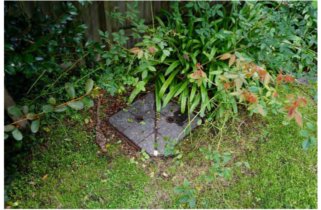
Figure 27 – Underground servicing at No. 4 Highgate Road.
