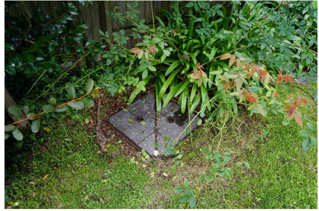
Figure 19 – Underground servicing at No. 4 Highgate Road.
