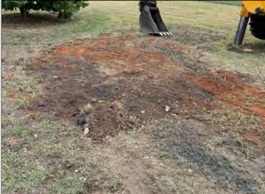
PHOTO 10: BACKFILL OF P_TP01 ALONG NORTHEASTERN BORDER OF THE SITE
