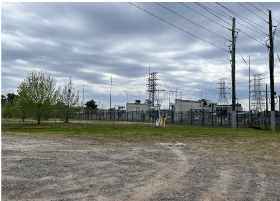
Figure 6-2: View of existing Penrith Substation infrastructure, looking southwest showing larger height compared to proposed new BESS elements (Aurecon 2024)
