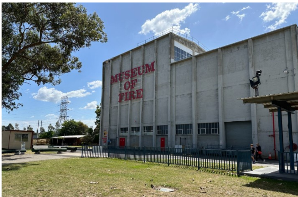
Figure 3-1: Museum of Fire, 1 Museum Drive (Aurecon, October 2024)
